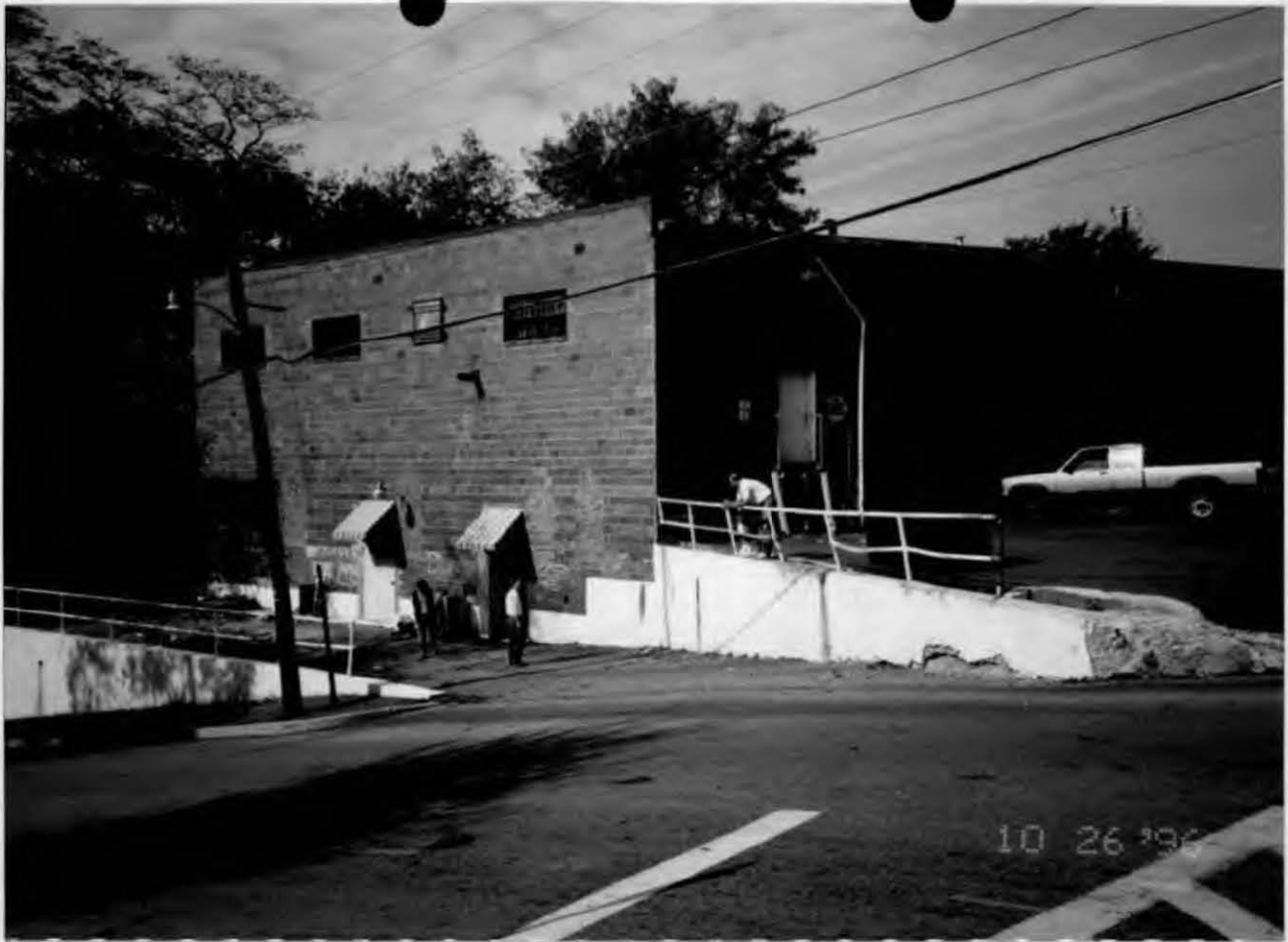
REAR OF STORE (SOUTH - FACING COLUMBIA AVE.) & PARTIAL EAST SIDE
