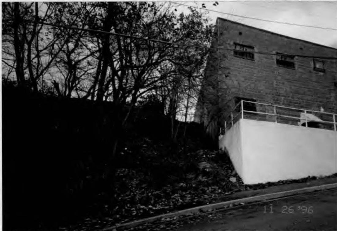
PARTIAL REAR (SOUTH) & PARTIAL WEST SIDE (FACING TAKOMA JUNCTION)
