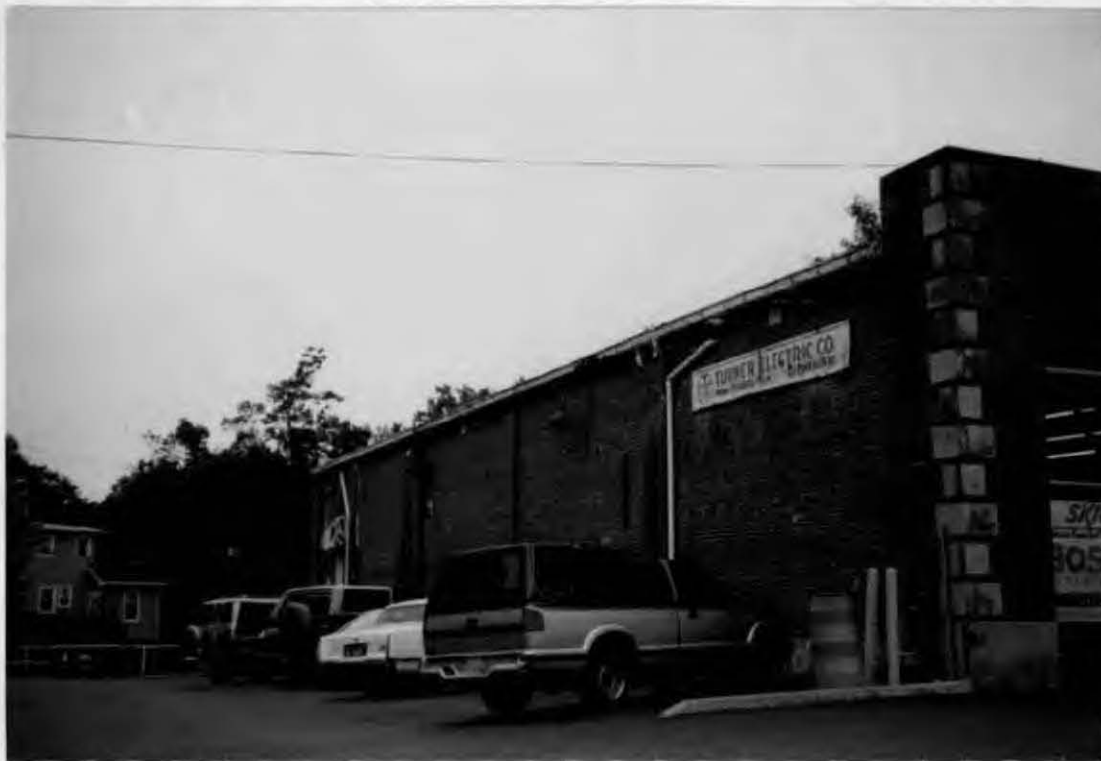
EAST SIDE OF STORE (FACING SYCAMORE AVENUE)
