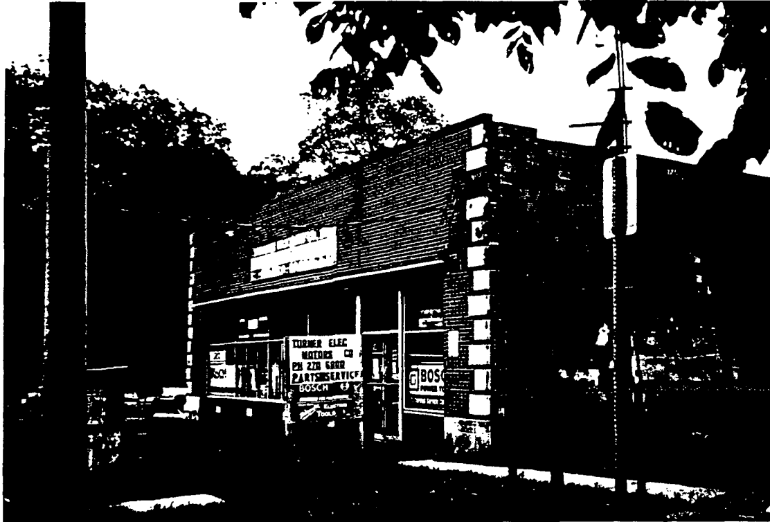
FRONT OF STORE (NORTH -FACING ETHAN ALLEN) AND PARTIAL R. WEST SIDE
