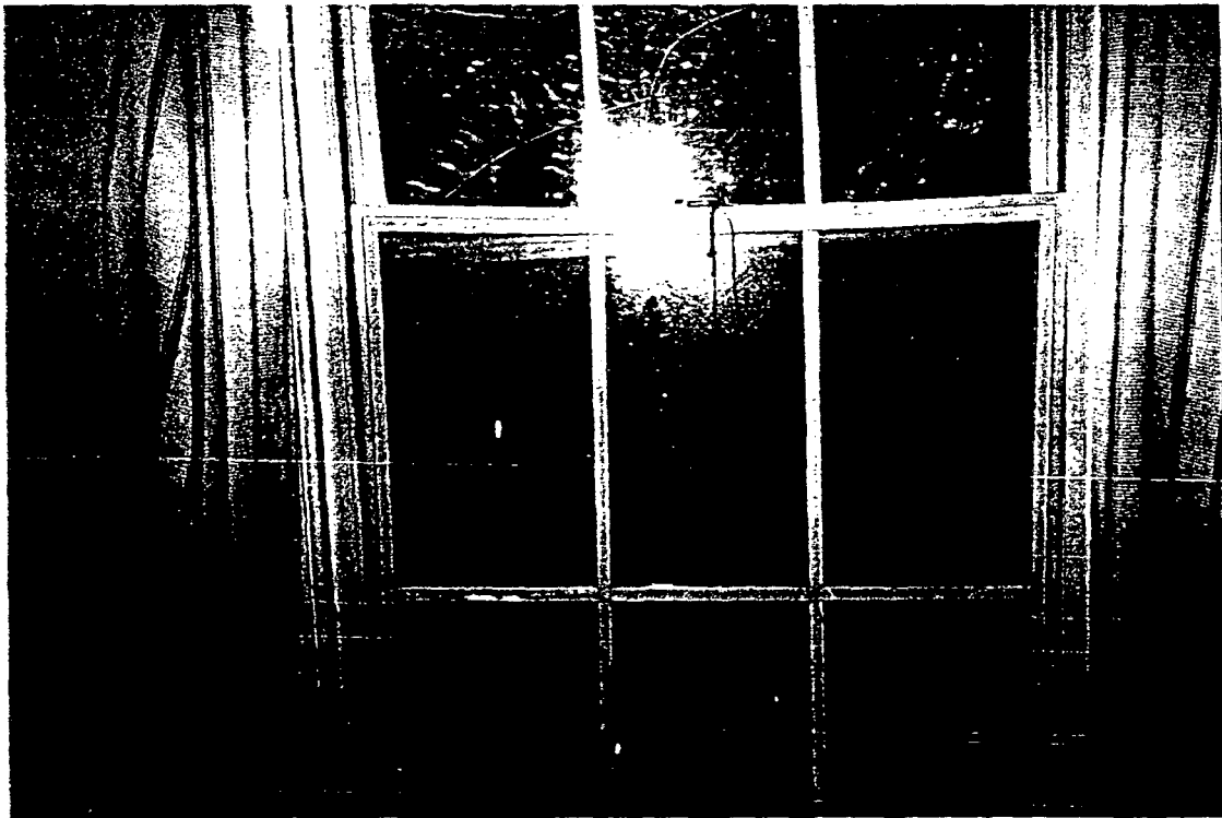
Distorted Window, wired together with coat hanger
