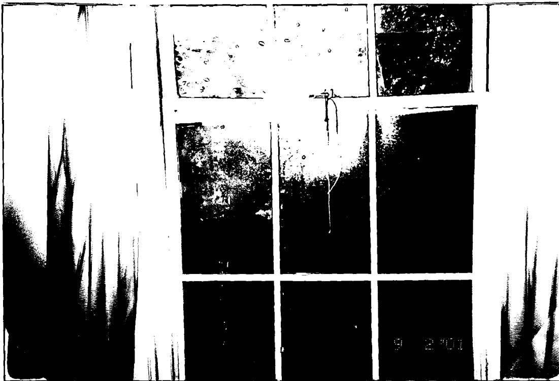
Distorted Window, wired together with coat hanger
