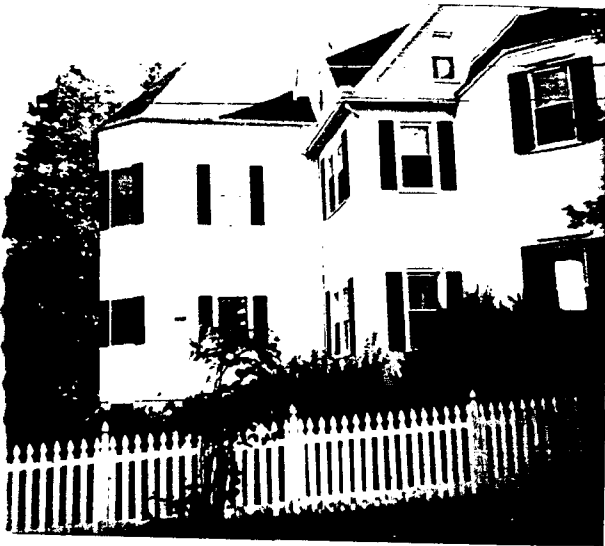
SOUTH SIDE 10300 FAWCETT ST KENSINGTON
