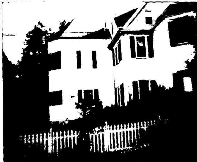
SOUTH SIDE 10300 FAWCETT ST KENSINGTON
