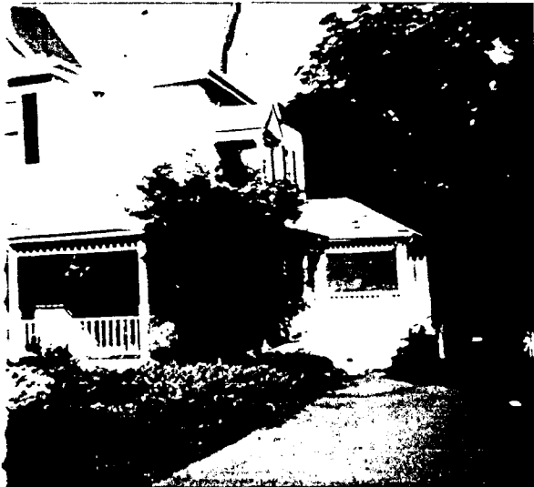
NORTH SIDE 10300 FAWCETT ST KENSINGTON
