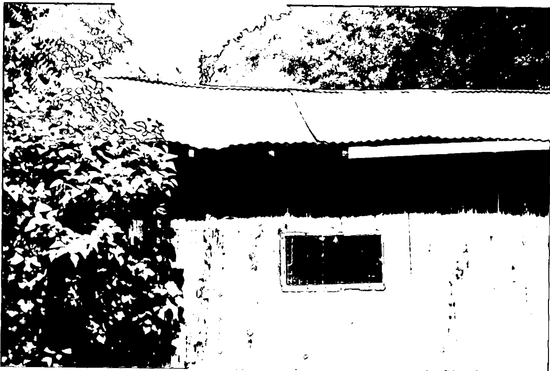
Roof falling apart, panels blow up in the air with good strong winds
