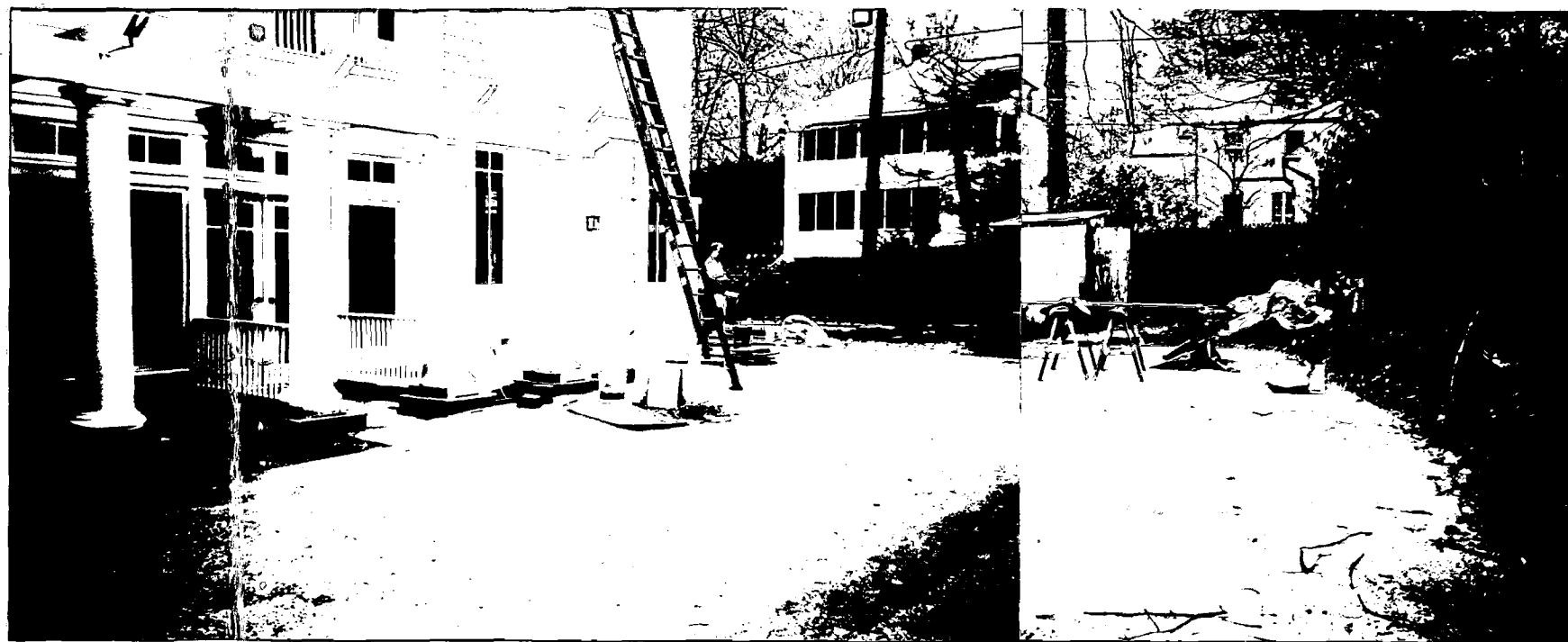
LOOKING SOUTH @ TERRACE, DRIVEWAY & GARAGE SITE
