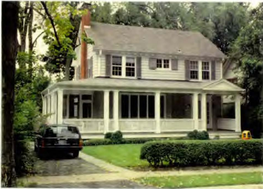
FRONT (VIEW FROM WEST IRVING)
