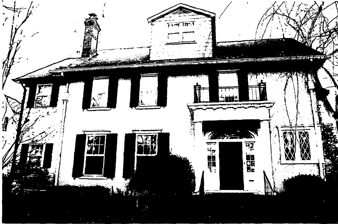
PHOTO OF EXISTING DORMER
