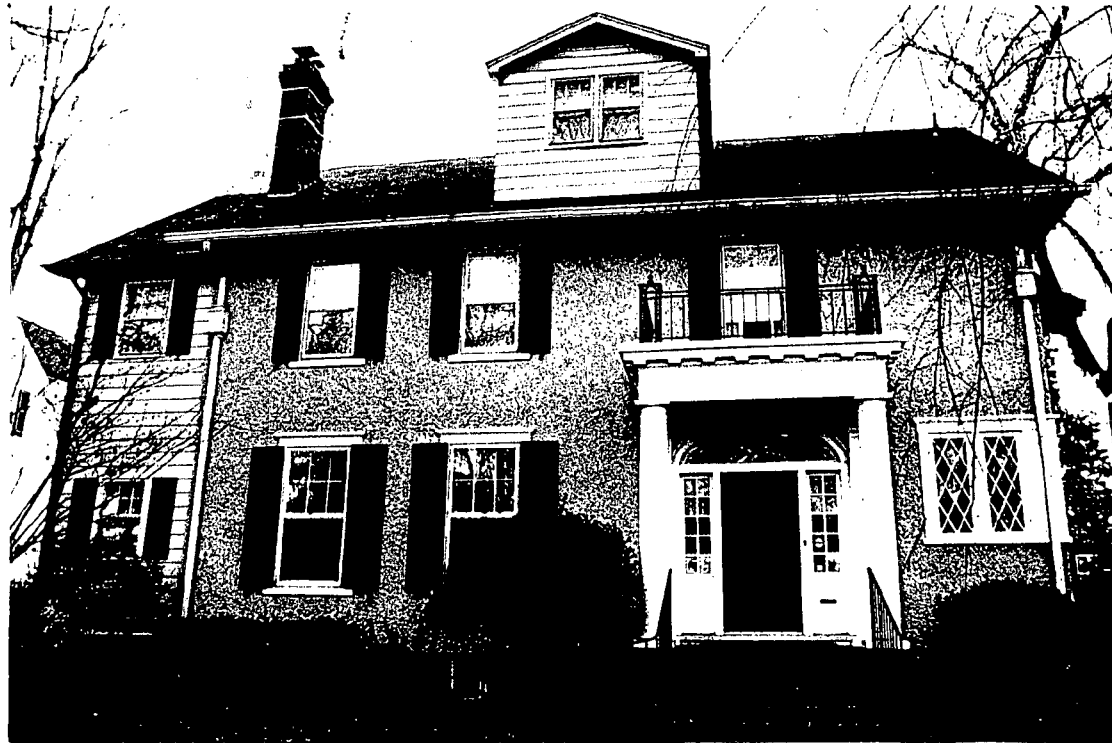
PHOTO OF EXISTING DORMER
