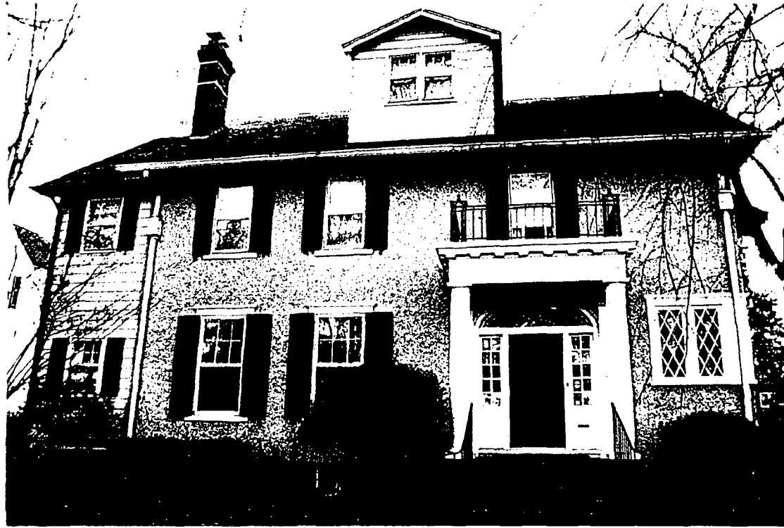
PHOTO OF EXISTING DORMER
