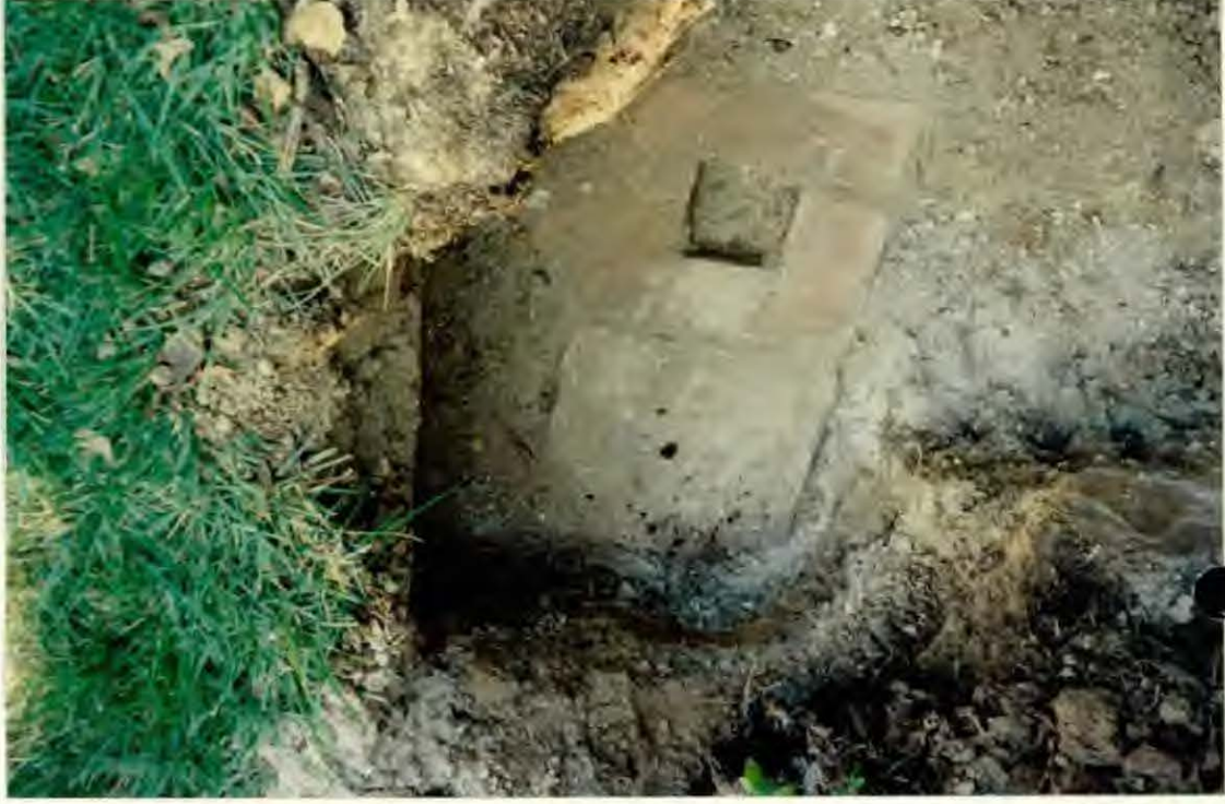
↗ Photo showing pier footings. Location: 9'-0" from face of building.
