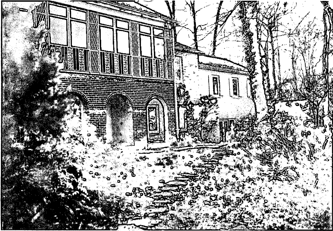
View of rear porch from South east
