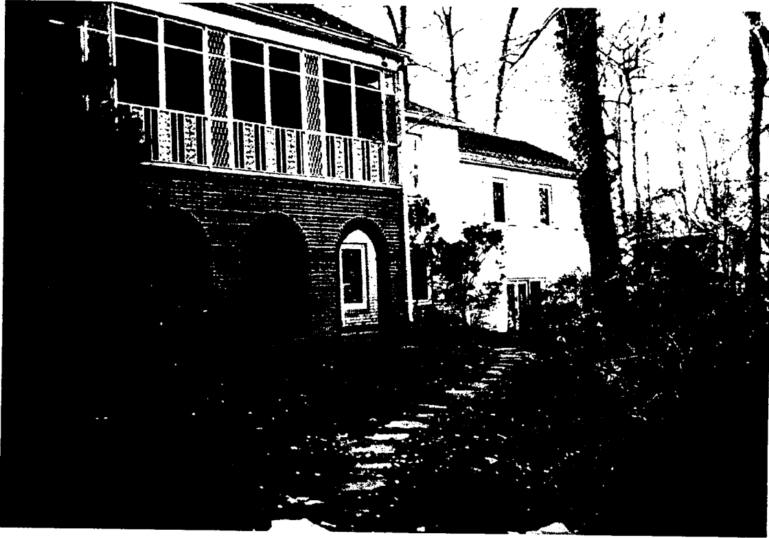
View of rear porch from South east
