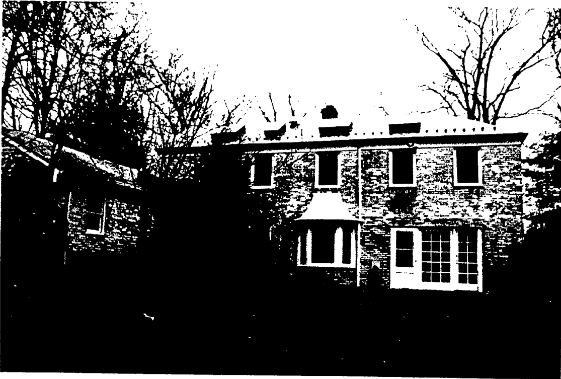
View of courtyard from South
