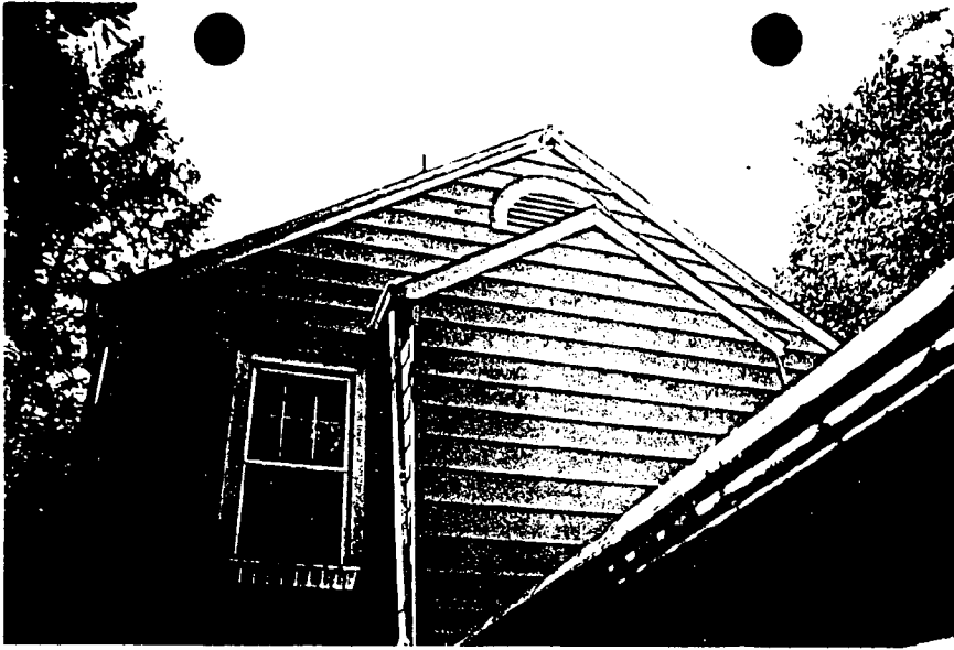
DETAIL OF REAR ROOF
