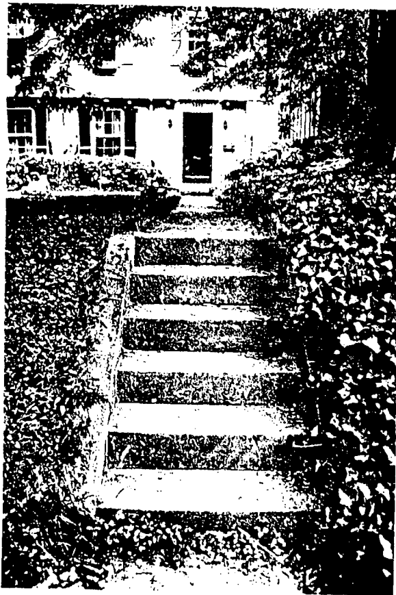
DETAIL OF FRONT OF HOUSE
