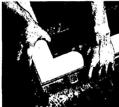
45° door and window mitering
