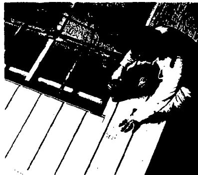
Wall Panel Jig for quality fit
