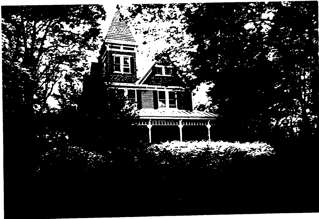
11018 Kenilworth Avenue before the fire
