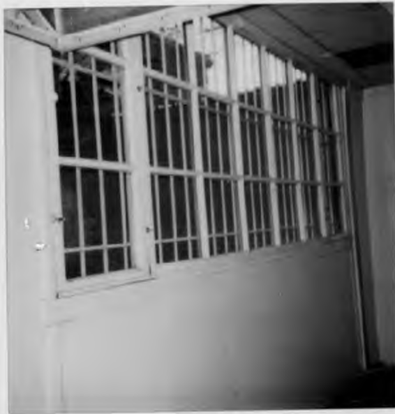
INTERIOR WINDOW - Cafe MORST DOOR TO WALL BACK
