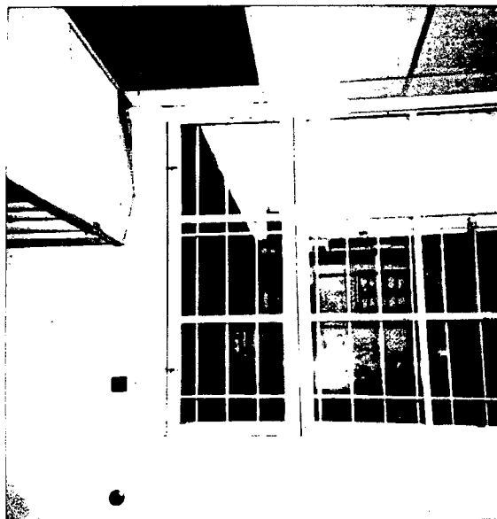
Window and ceiling - Cafe Monet (looking out to courtyard)
