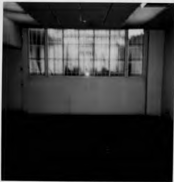
INTERIOR WINDOW WALL FACADE - CAFE MONST
