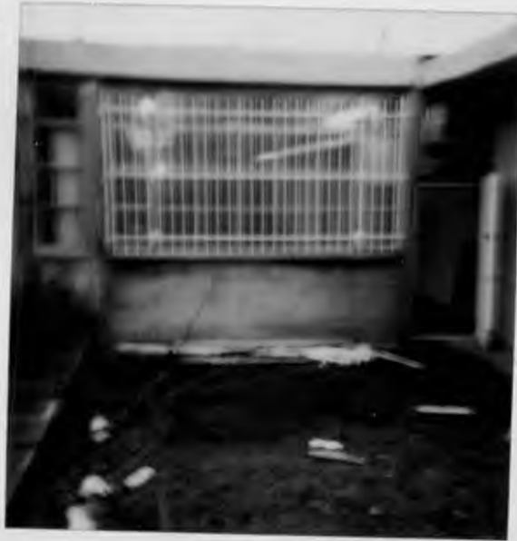
COURTYARD LOOKING - CARO MOUNT TO WINDOW WALL
