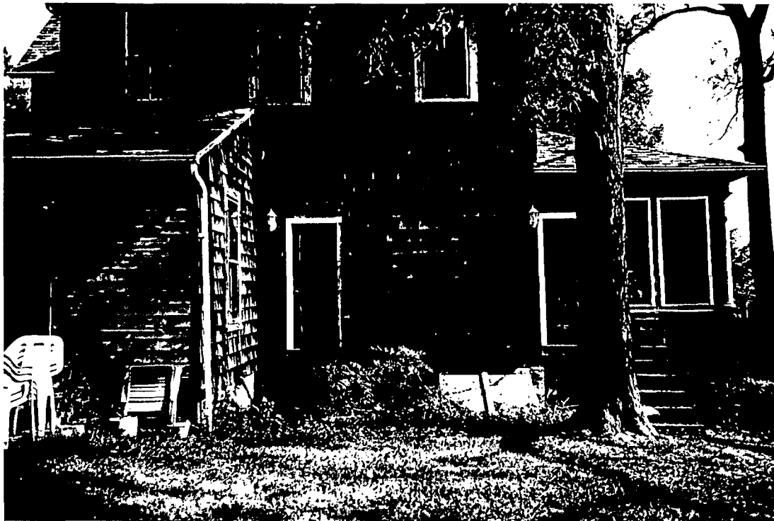
Rear SIDE VIEW (EAST) FROM CONNECTICUT AVENUE SHOWING ENCLOSED PORCH, SIDE OF SHED ADDITION, WALNUT TREE AND SPACE FOR NEW DECK
