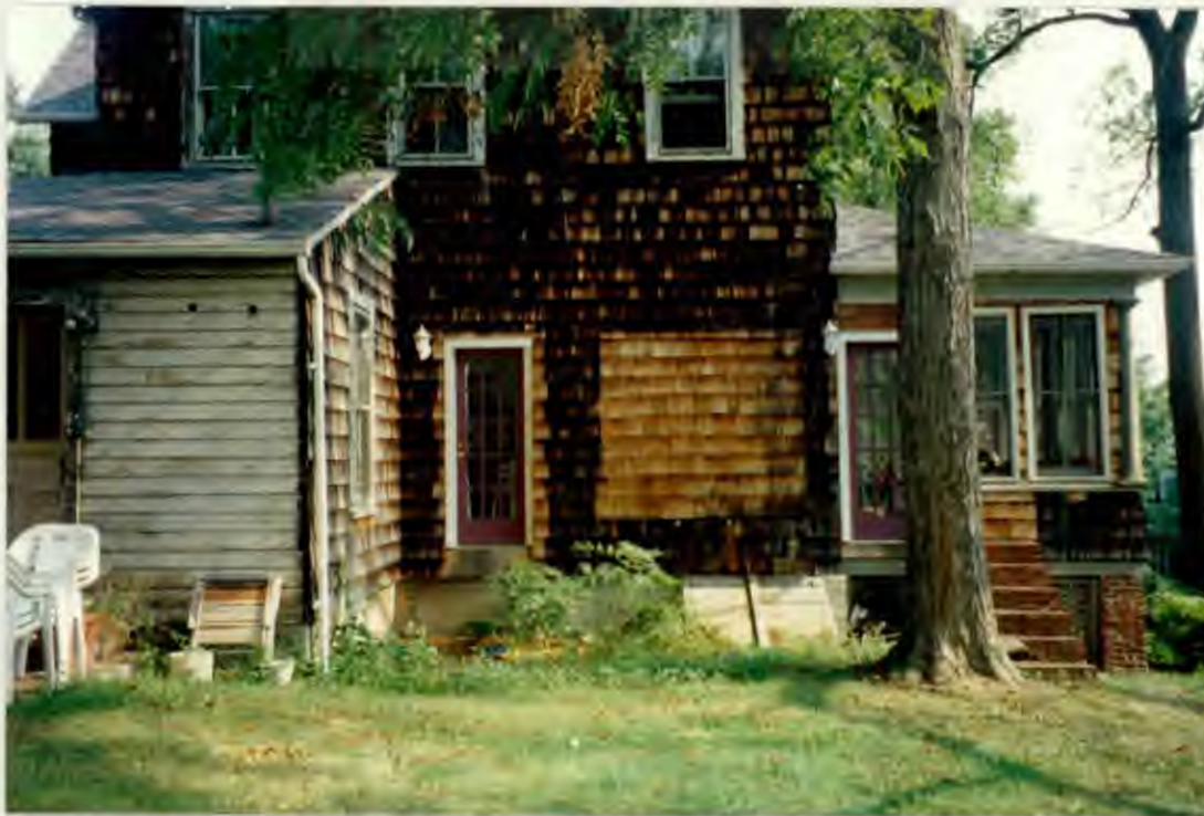
Real SIDE VIEW (EAST) FROM CONNECTICUT AVENUE SHOWING ENCLOSED PORCH, SIDE OF SHED ADDITION, WALNUT TREE AND SPACE FOR NEW DECK
