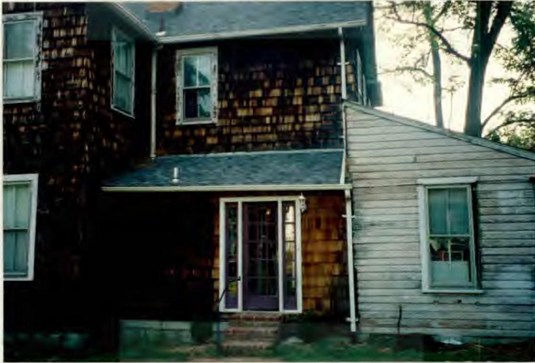
WEST SIDE VIEW SHOWING SHINGLES AND ORIGINAL SIDING WHERE SHINGLES REMOVED
