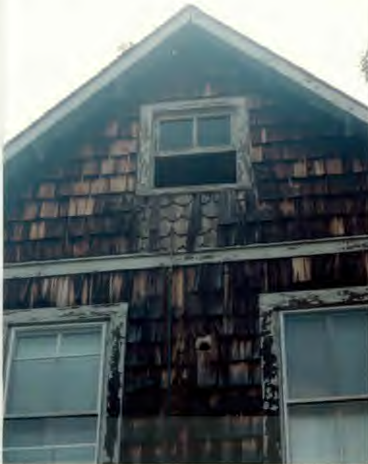
CLOSE UP OF GABLE SHOWING DECORATIVE SHINGLES
