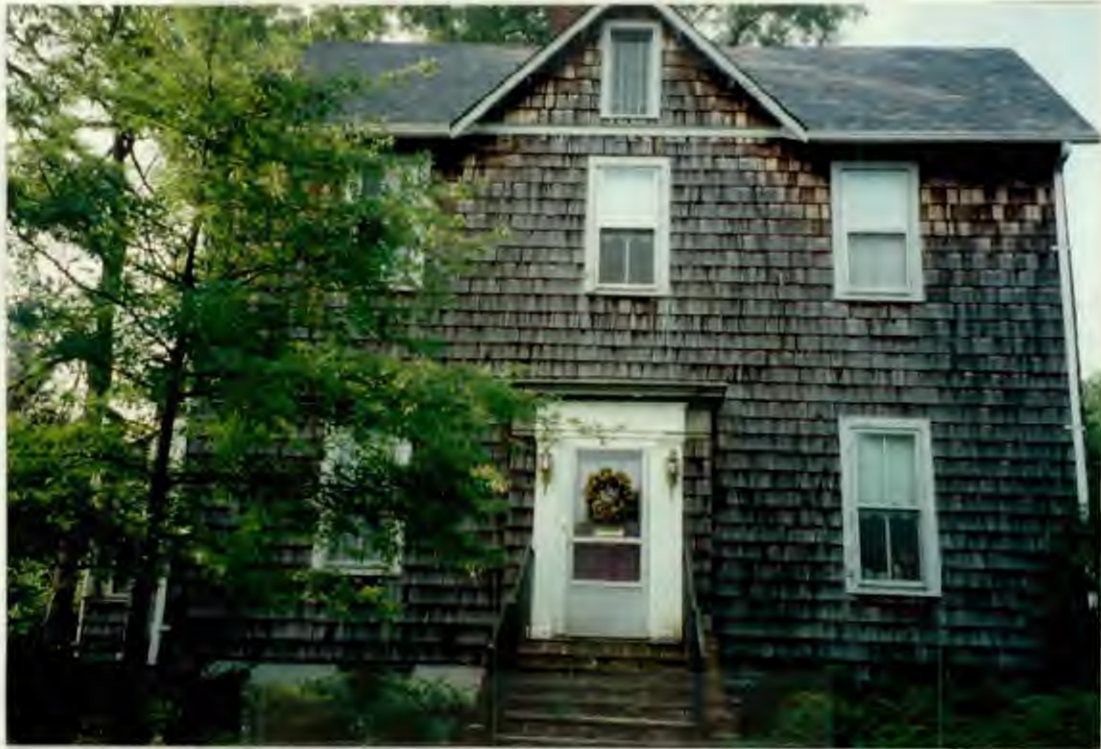
FRONT VIEW FACING BALTIMORE STREET
