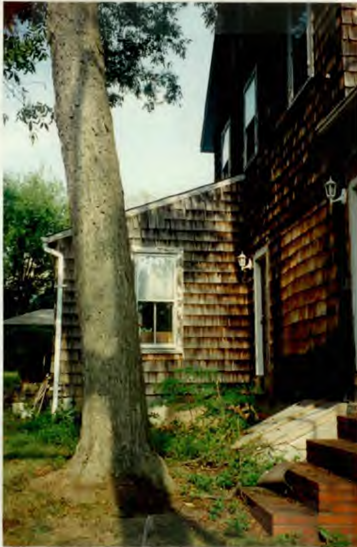
CLOSE UP OF AREA WHERE DECK WILL BE LOCATED
