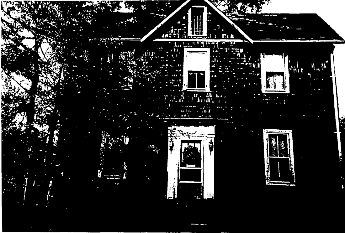
FRONT VIEW FACING BALTIMORE STREET
