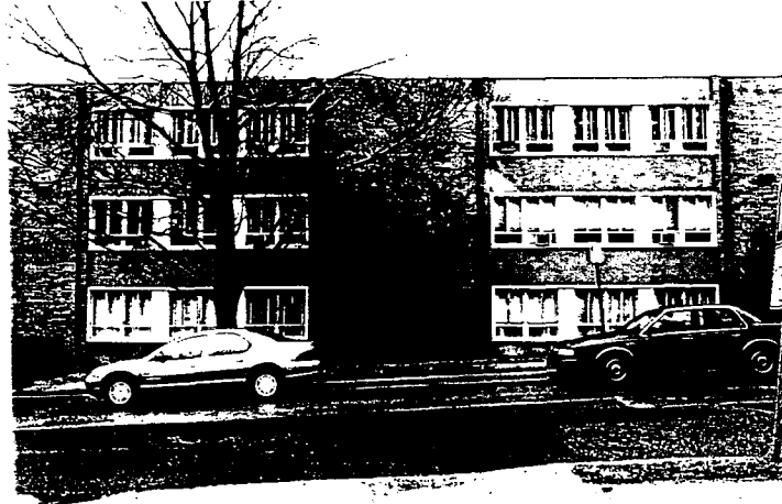
PRIMARY EXTERIOR WORK AREA - NEW LOUVERS BELOW WINDOWS. REMOVE AC UNITS
