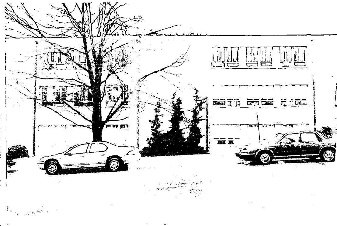
PRIMARY EXTERIOR WORK AREA - NEW LOUVERS BELOW WINDOWS, REMOVE AC UNITS
