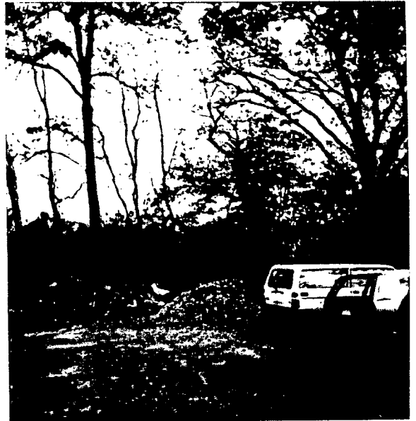
NEW SHED WILL BE BETWEEN HICKORY AND OAK WHERE WOODCHIP PILE IS IN PICTURE
