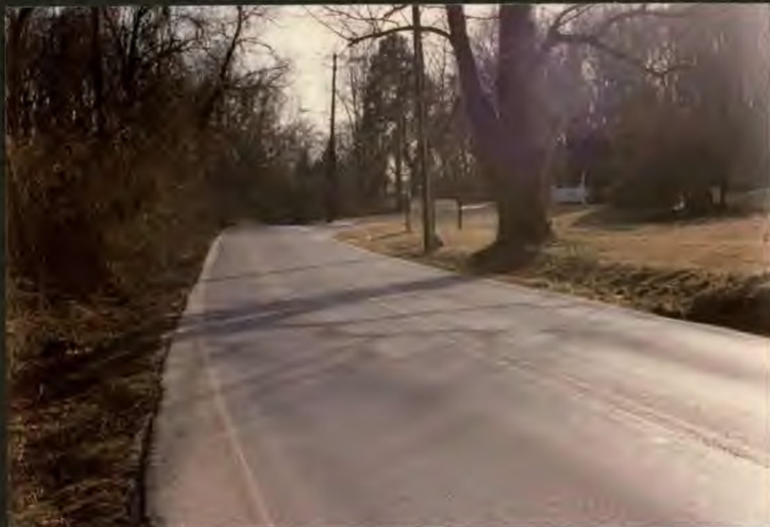
Looking south; photo taken from ANS property across the street, close to 9001 Jones Mill Rd.
