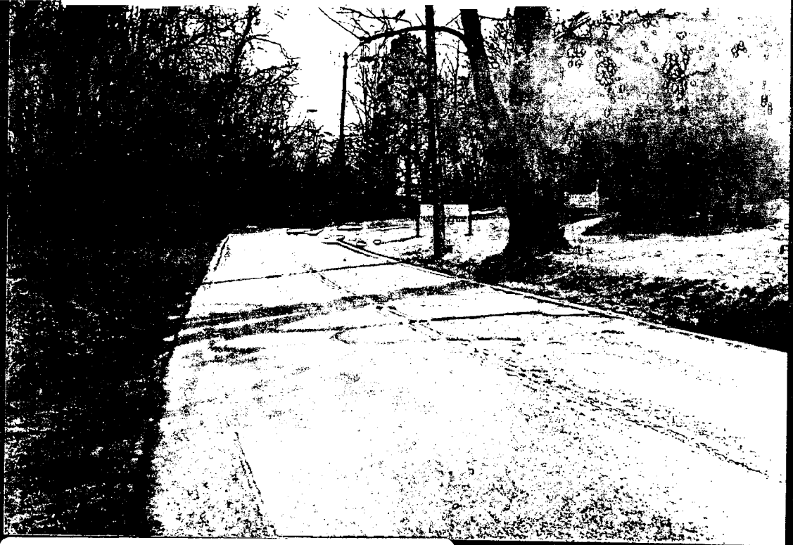
Looking south; photo taken from ANS property across the street, close to 9001 Jones Mill Rd.
