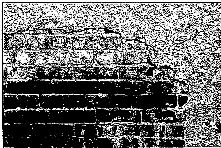
Detail of Chevy Chase Club Carriage House wall with pebble-dash stucco and American bond brick.
