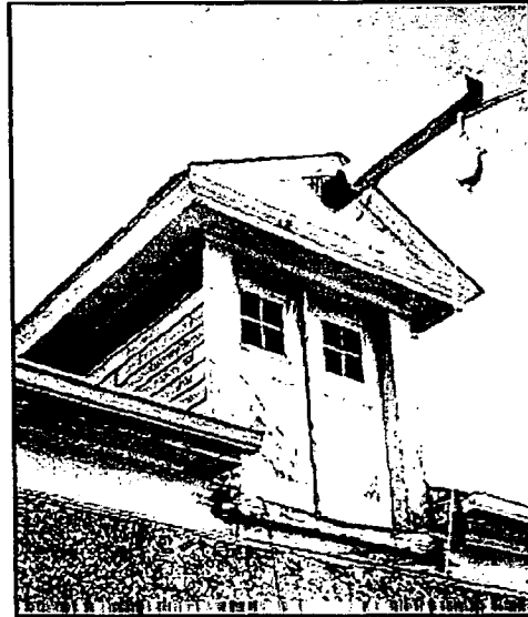
Detail of original hay loft doors at north elevation of the Chevy Chase Club Carriage House. Source: Robinson & Associates
