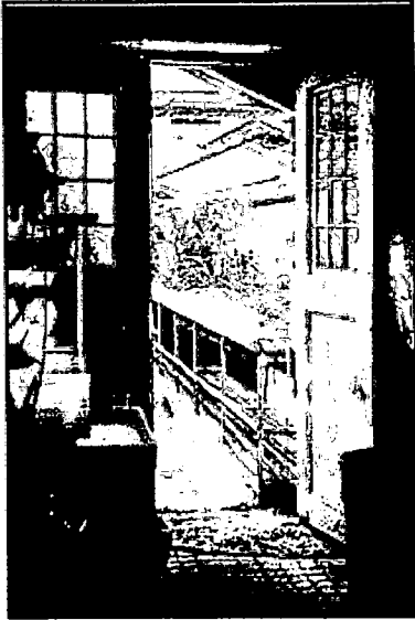
Detail of original stable door at greenhouse entrance (South facade) of the Chevy Chase Club Carriage House. Source: Robinson & Associates
