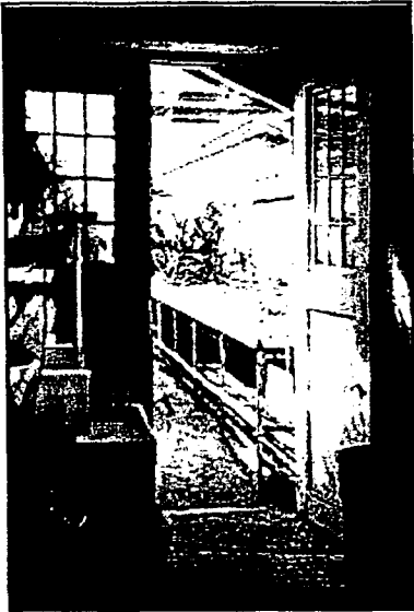
Detail of original stable door at greenhouse entrance (South facade) of the Chevy Chase Club Carriage House. Source: Robinson & Associates
