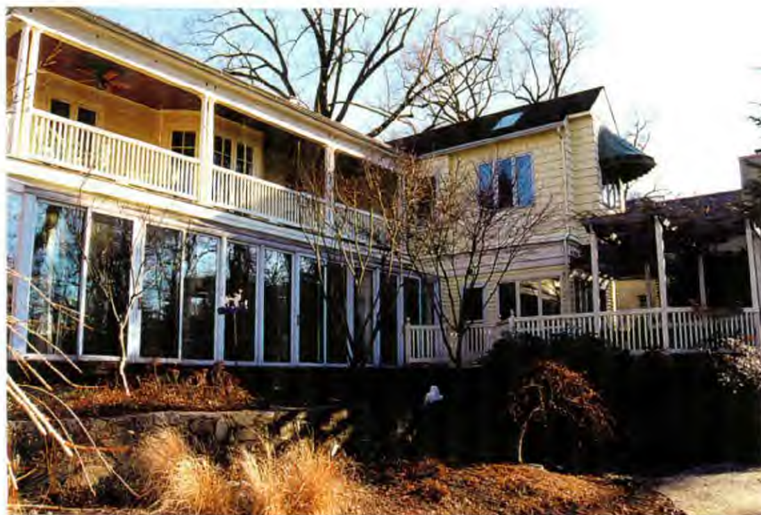
Rear Elevation - Area of Addition
