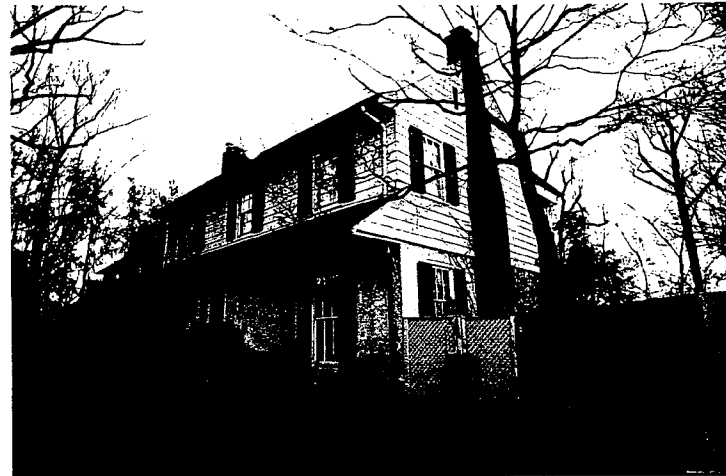
Front Elevation - Area of Addition
