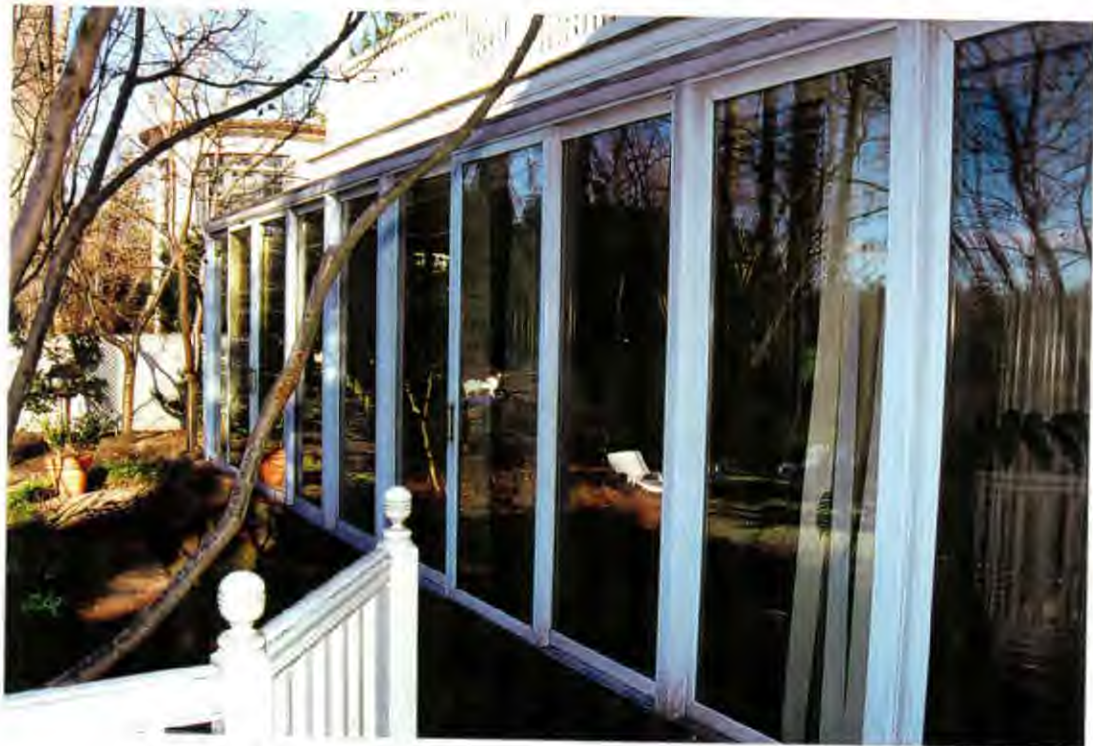
Rear Elevation - Area to be Removed
