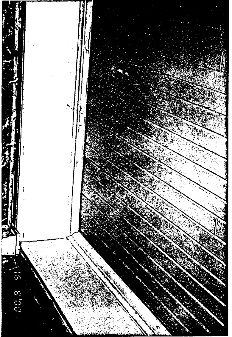
INTERIOR WOOD CEILING
