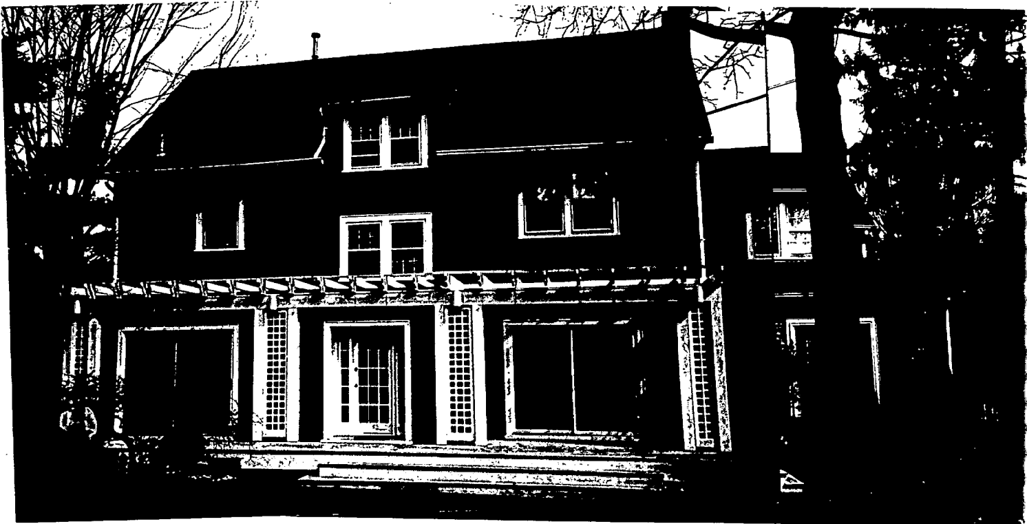
REAR VIEW: SOUTH SIDE ↑
