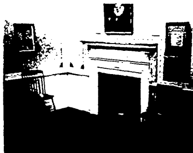
Figure 2. The paint chronology of this mantel, seen in the exposed paint layers in the left corner, proved it had been relocated from another room of the house. To restore a significant feature's paint history and the mantel to its original sequence or color by stripping off all the paint is inappropriate — and unnecessary — as part of a lead hazard reduction project. Careful surface preparation and repainting with lead-free top coats are recommended. Photo: NPS Files.
