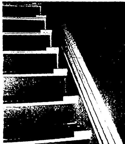
Figure 21. Painted stairs and floors can cause a problem because lead dust settles between the wooden boards. In this case, the steps were sanded, repainted, and covered with rubber stair treads. The floors could not be effectively cleaned and sealed so they were isolated with a new subflooring, and a washable tile finish installed.
