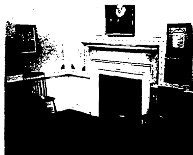
Figure 2. The paint chronology of this mantel, seen in the exposed paint layers in the left corner, proved it had been relocated from another room of the house. To remove a significant feature's paint history and the evidence of its original sequence of color by stripping off all the paint is inappropriate — and unnecessary — as part of a lead hazard reduction project. Careful surface preparation and repainting with lead-free top coats is recommended. Photo: NPS Files.
