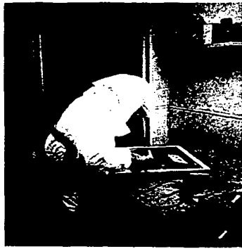
Low-level heat guns can be used to remove lead-based paint from significant historic windows and trimwork, but a worker exposed to lead dust over an extended period of time must be protected from the hazards created during the process of paint removal. Photo: Williamsport Preservation Training Center.
