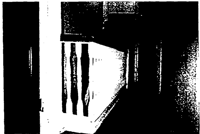
Figure 28. This recently completed housing, which is now lead-safe, could become re-contaminated from lead in air if children are not maintained. Damp mopping floor surfaces and regular dusting to keep the house clean will ensure its continuing safety.
