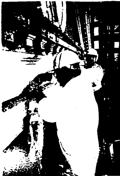
Figure 10. The choice of paint removal method will trigger various environmental controls and worker protection. The chemical poultice-type paint remover uses a paper backing that keeps the lead waste contained for proper disposal. The worker is adequately protected by a suit and gloves; for this work a respirator tests not required. Local laws required containment and neutralization of any after-wash water run off. Photo: NPS Files.
