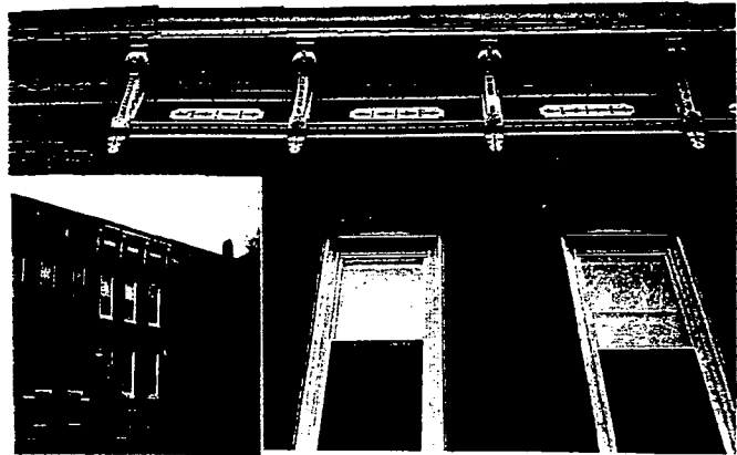
Figure 18. As part of an urban housing grant program, the exterior of this row house was successfully made lead-safe and met the Secretary of the Interior's Standards for Rehabilitation. The exterior was washed, then repainted with exterior grade alkyd paint. The decorative roof brackets and cornice were repainted; not removed or covered as is often recommended in typical abatement guidelines. The previously altered, deteriorated window sash were replaced with new sash and jamb liners set within the historic frames. Photos: Deborah Birch.
