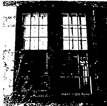
Figure 6. Deteriorating operable windows often contribute to lead dust in a house. Peeling paint and small particles from abraded surfaces collect in window troughs or sills and are then carried inside by air currents, settling on floors. When the lead dust mixes with regular house dust, it can easily be ingested by a child through hand-to-mouth contact. In homes with small children, floors and other surfaces should be kept as clean as possible to avoid lead contamination.
