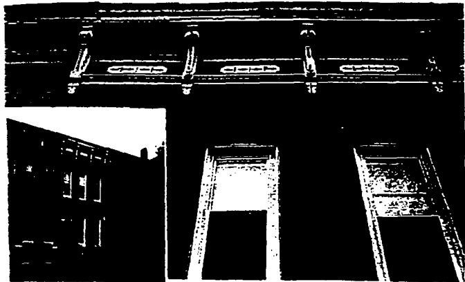
Figure 18. As part of an urban housing grant program, the exterior of this row house was successfully made lead-safe and met the Secretary of the Interior's Standards for Rehabilitation. The exterior was washed, then repainted with exterior grade alkyd paint. The decorative roof brackets and cornice were repainted; not removed or covered as is often recommended in typical abatement guidelines. The previously altered, deteriorated window sash were replaced with new sash and jamb liners set within the historic frames. Photos: Deborah Birch.
