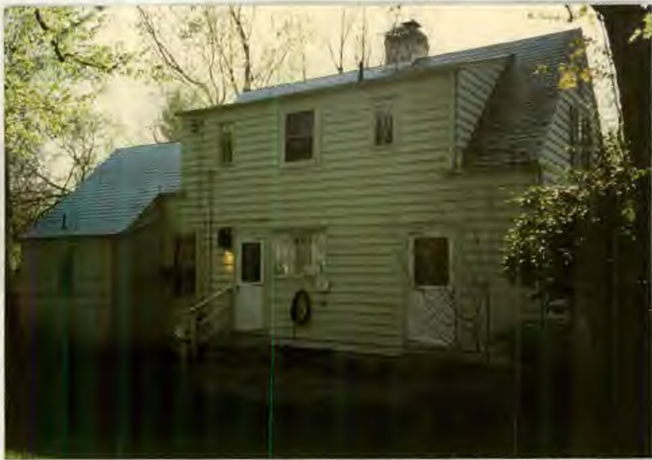
EAST ELEV (REAR) SHOWING NORTH FACADE
