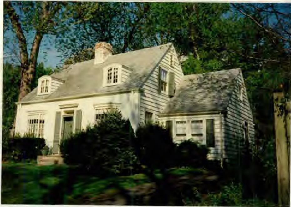
SHOWING SOUTH FACADE
