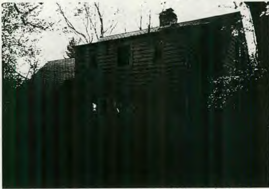
EAST ELEV (REAR) SHOWING NORTH FACADE
