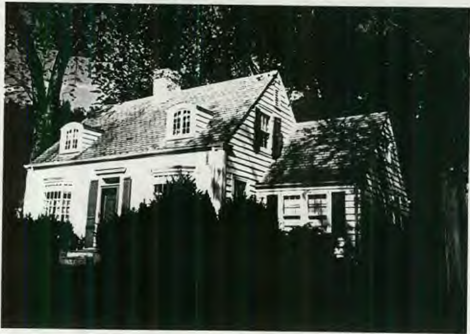
SHOWING SOUTH FACADE
