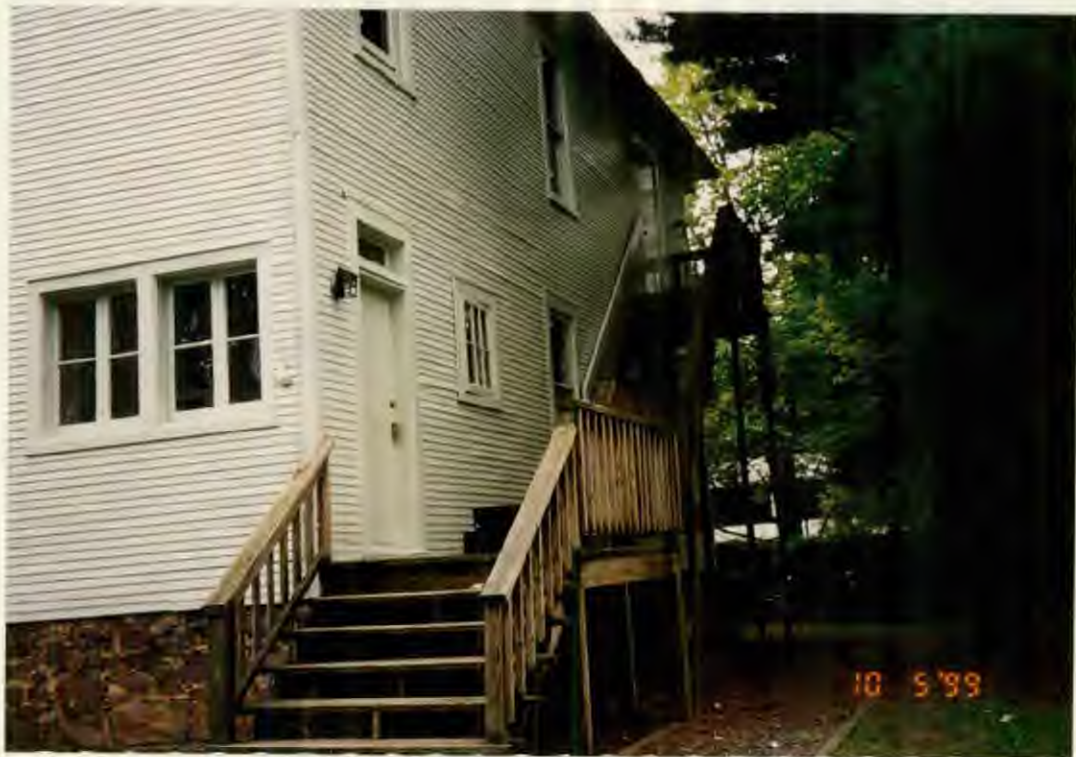
REAR VIEW- DECK(S) TO BE REMOVED
