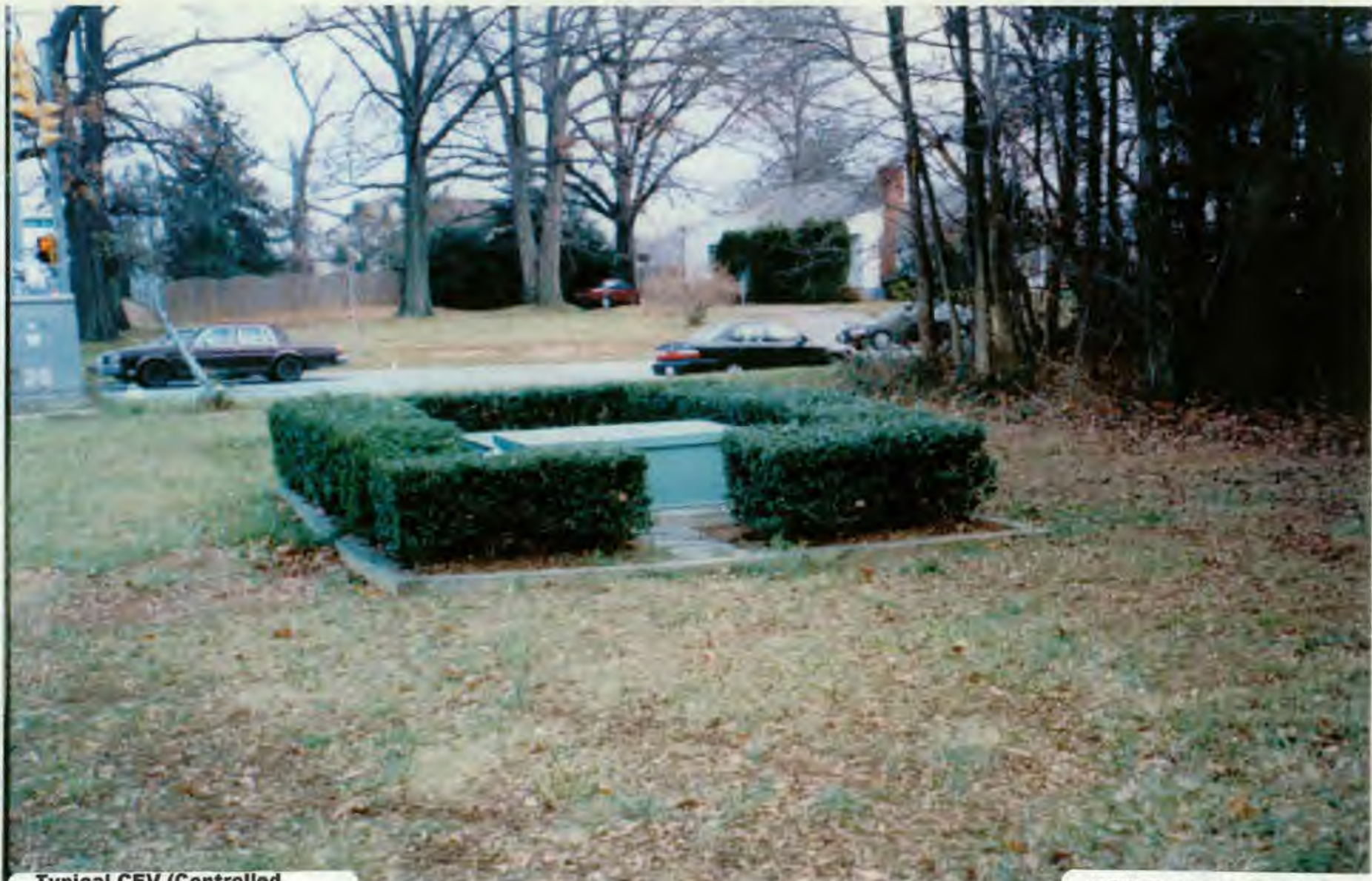
Typical CEV (Controlled Environmental Vault) – Shown with approx. 2 years shrubby growth
