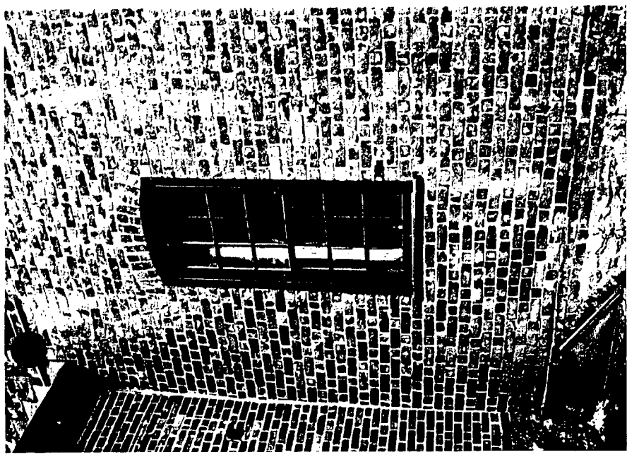
Window on North wall after restoration
