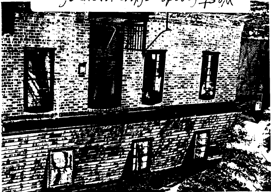
West facade after repair of brickwork and installation of copper guttering.
