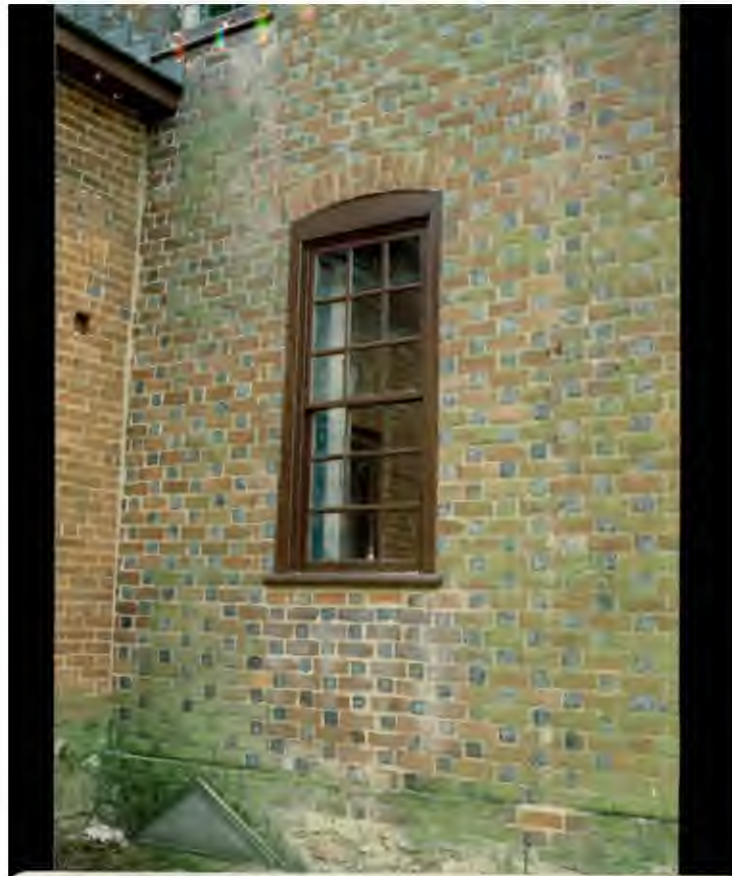
Window on North wall after restoration
