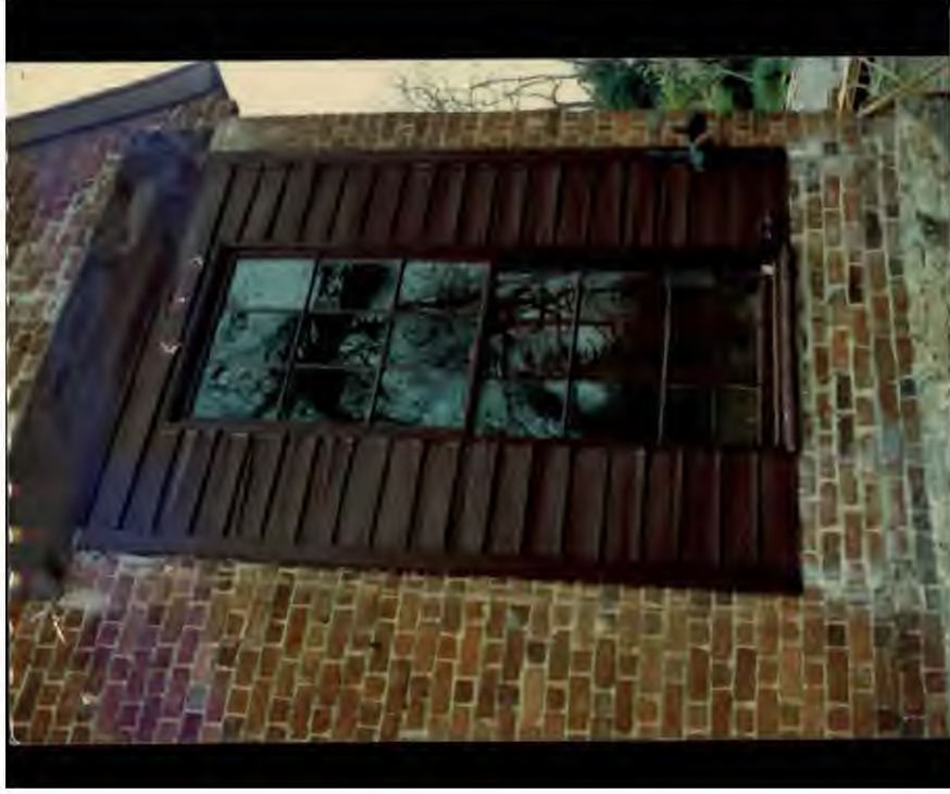
Window on south wall before restoration.
