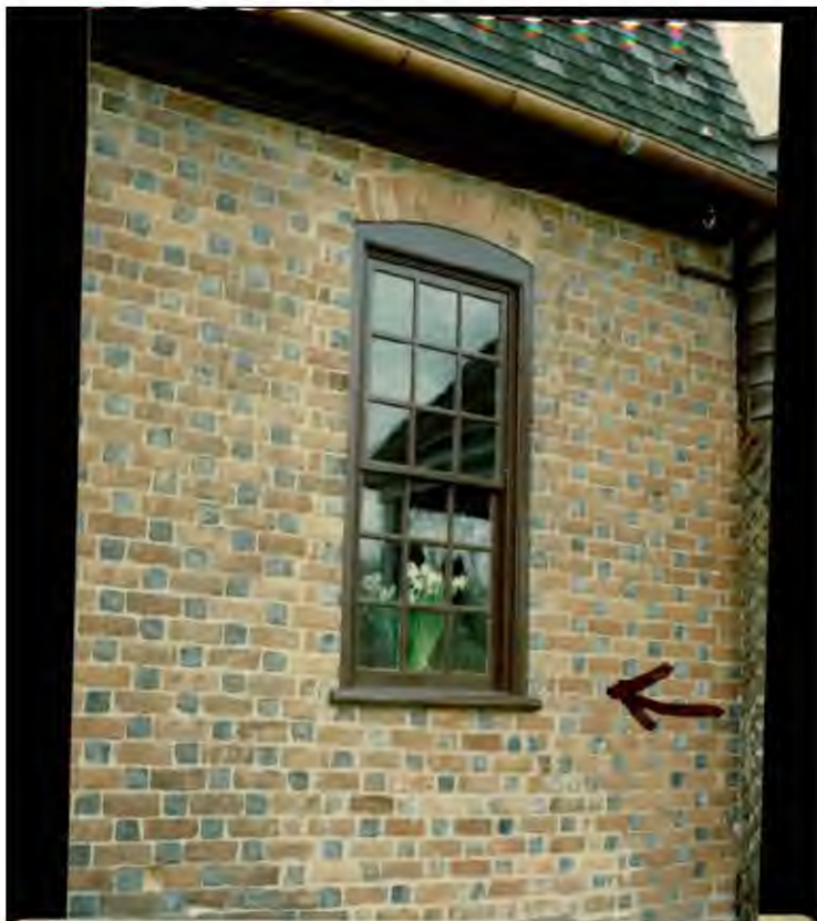
After restoration - Window #1 East facade, north window N.E
