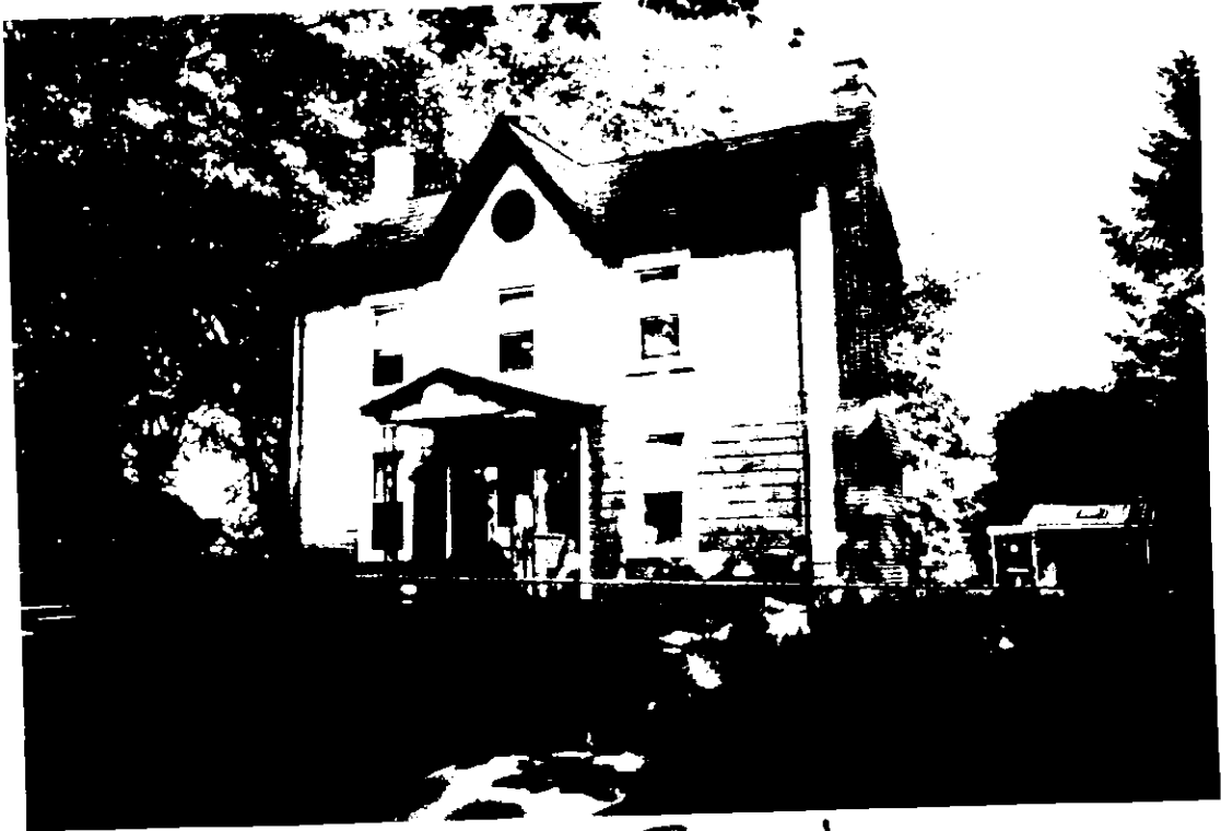
19925 White Ground Road Facade
