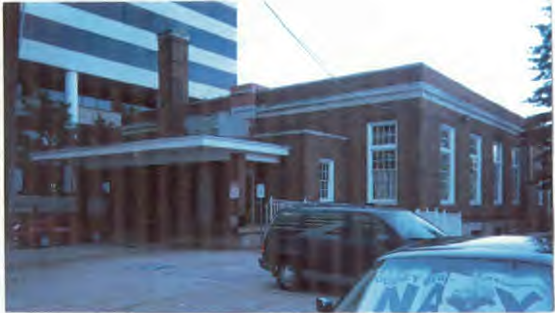
Above: View from southwest of alley
