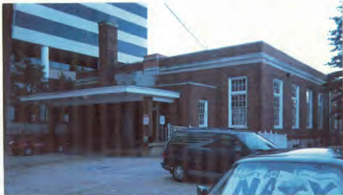
Above: View from southwest of alley
