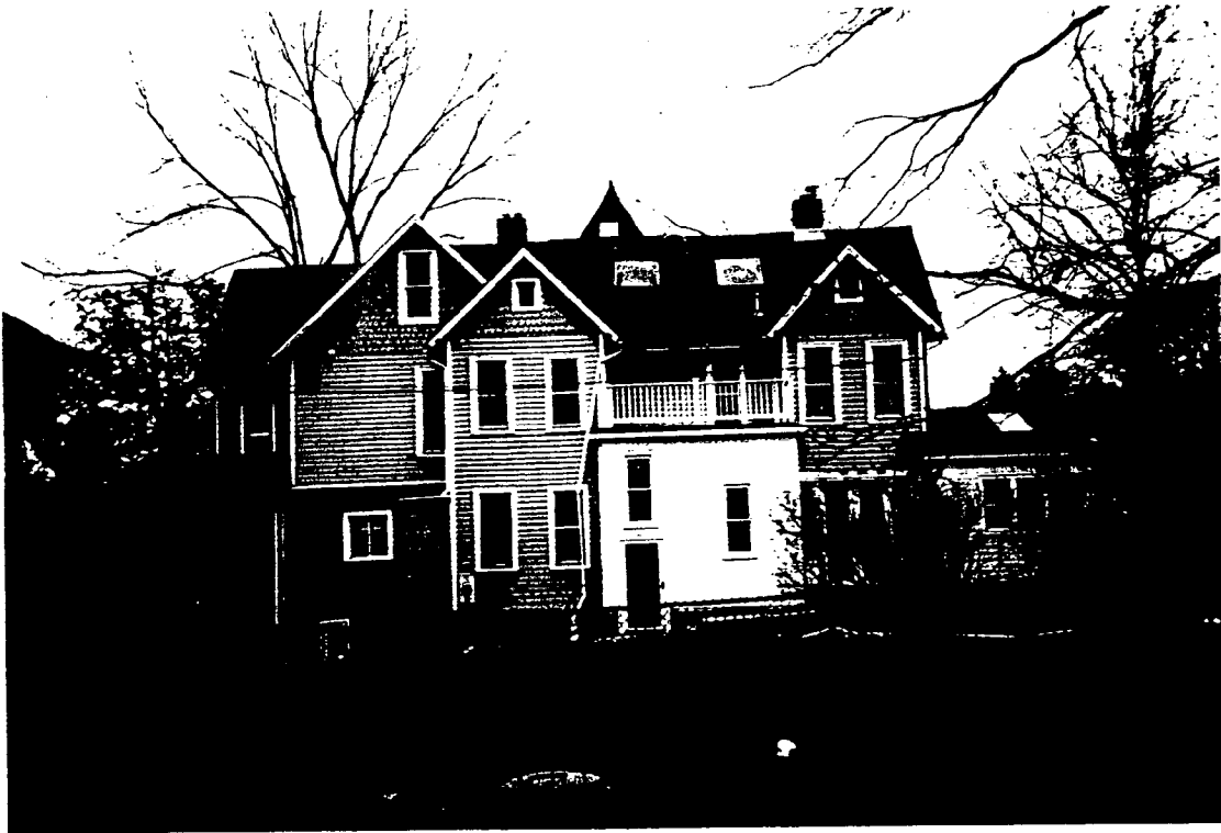
Rear property line. Side facade
