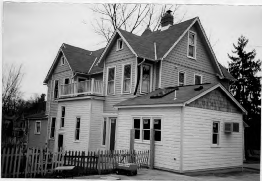
Rear Facade, 7300 7300 Baltimore Ave.
