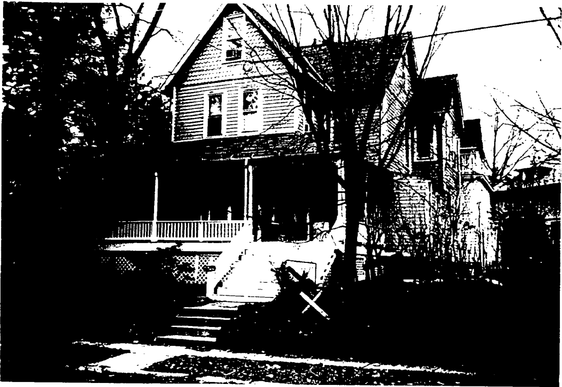
Baltimore Ave Facade
