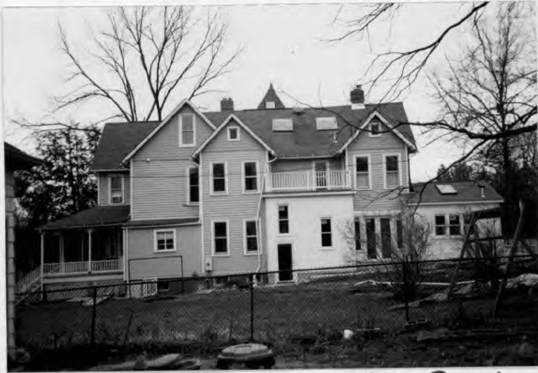
Rear property line. Side facade
