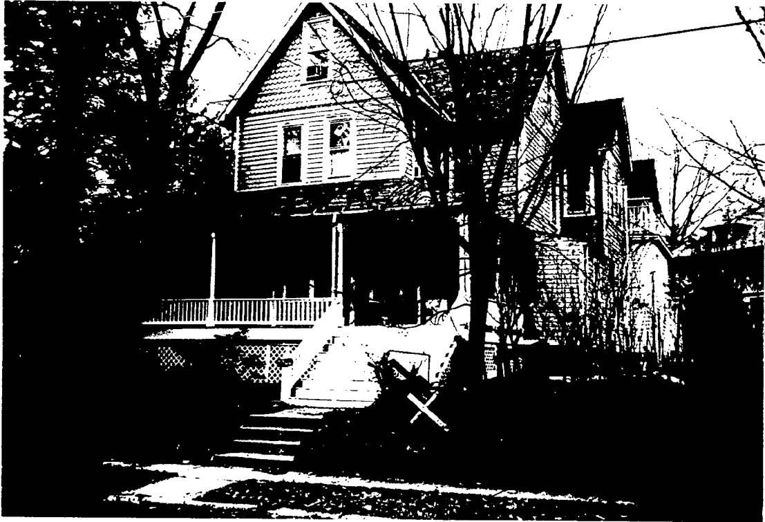
Baltimore Ave Facade
