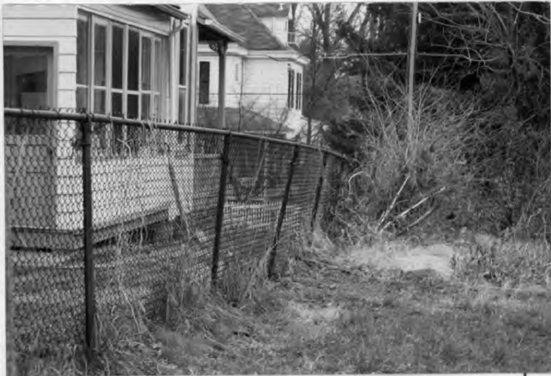
Existing fence on rear property line
