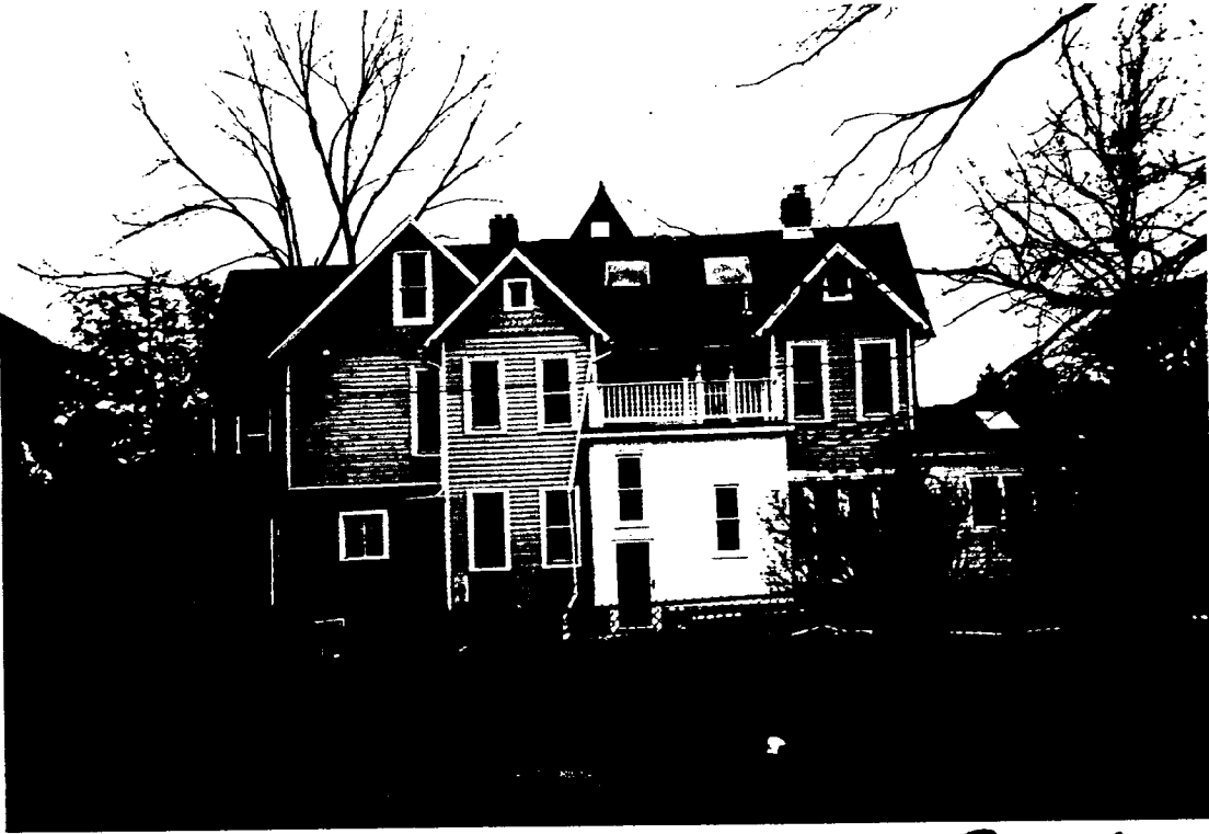
Rear property line. Side facade
