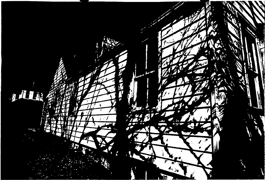
REAR CORNER - BUREAU SIDE
