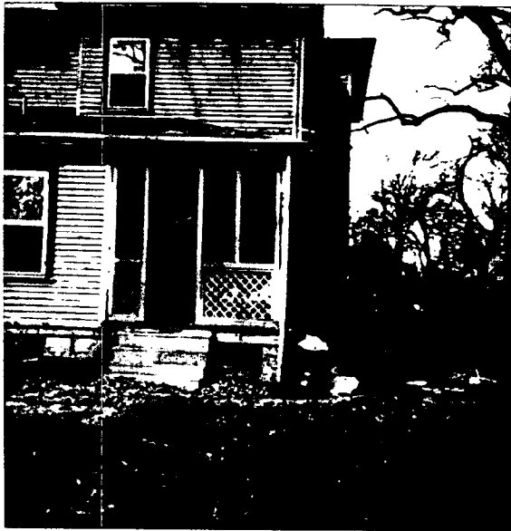
rear view of porch
