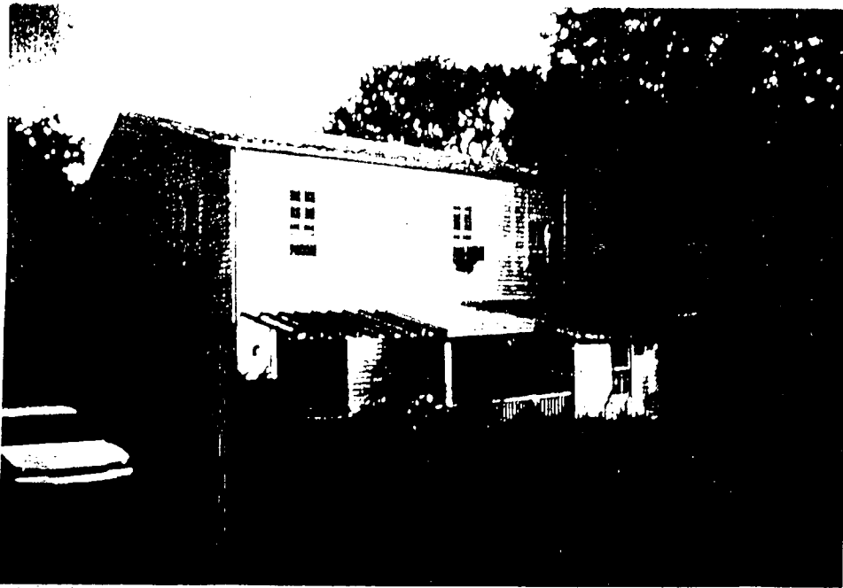
(15) existing house - rear view
