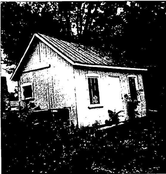
C. BROWNING FARM AT LITTLE BENNETT GOLF SMALL GARAGE TO BE DEMOLISHED APPROX. 10' x 12'. POTOMAC EDISON TRANSFORMER + C+P PEDUSTAL BETWEEN SHEDS
