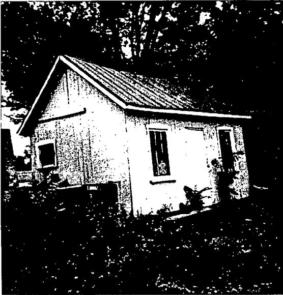
C. BROWNING FARM AT LITTLE BENNETT GOLF SMALL GARAGE TO BE DEMOLISHED APPROX. 10' x 12'. POTOMAC EDISON TRANSFORMER + C+P PIEDestal BETWEEN
