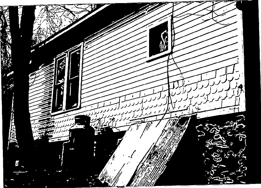
Trees needing to be removed that are damaging foundation,
