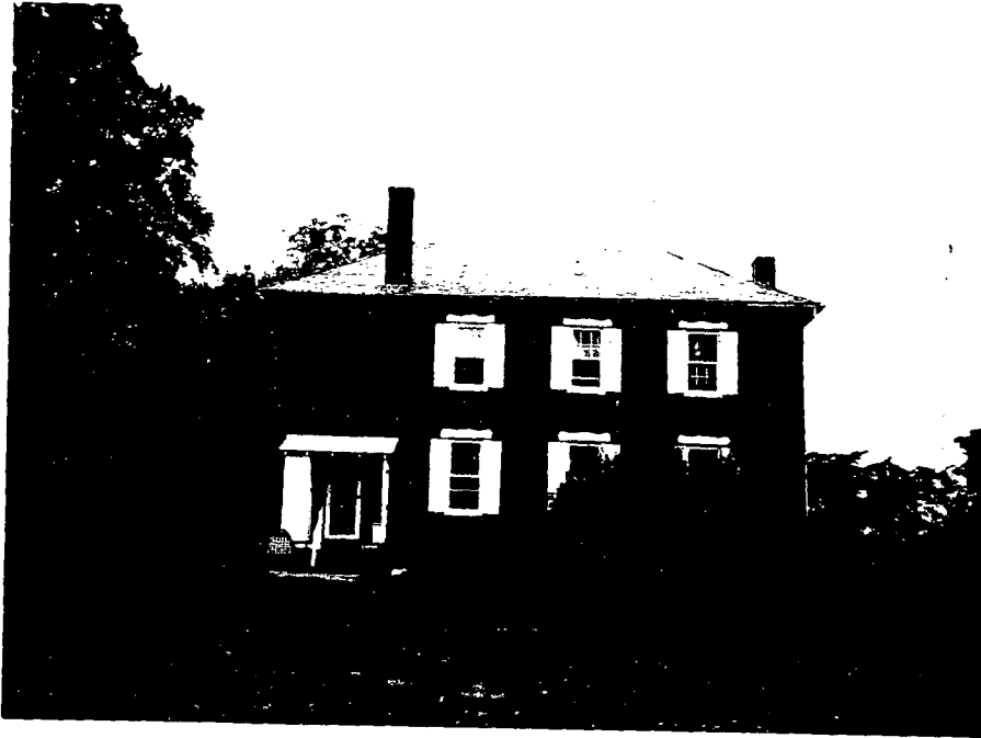
A - North Facade & Side Entrance of Main House - (Note numerous cracked slates)
