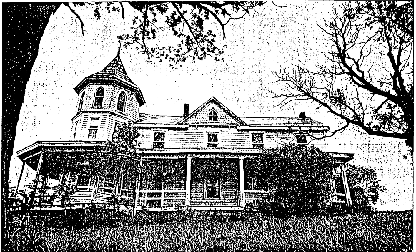
Renovation of the rambling mid-19th century Oliver Watkins farmhouse would be ideal for a group who can donate time and materials. Staff photo by Janet Worne
