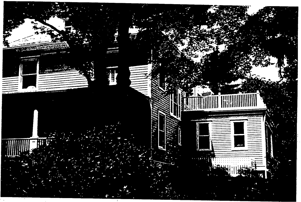
Side Addition- Capron House, Montgomery Avenue, Kensington
