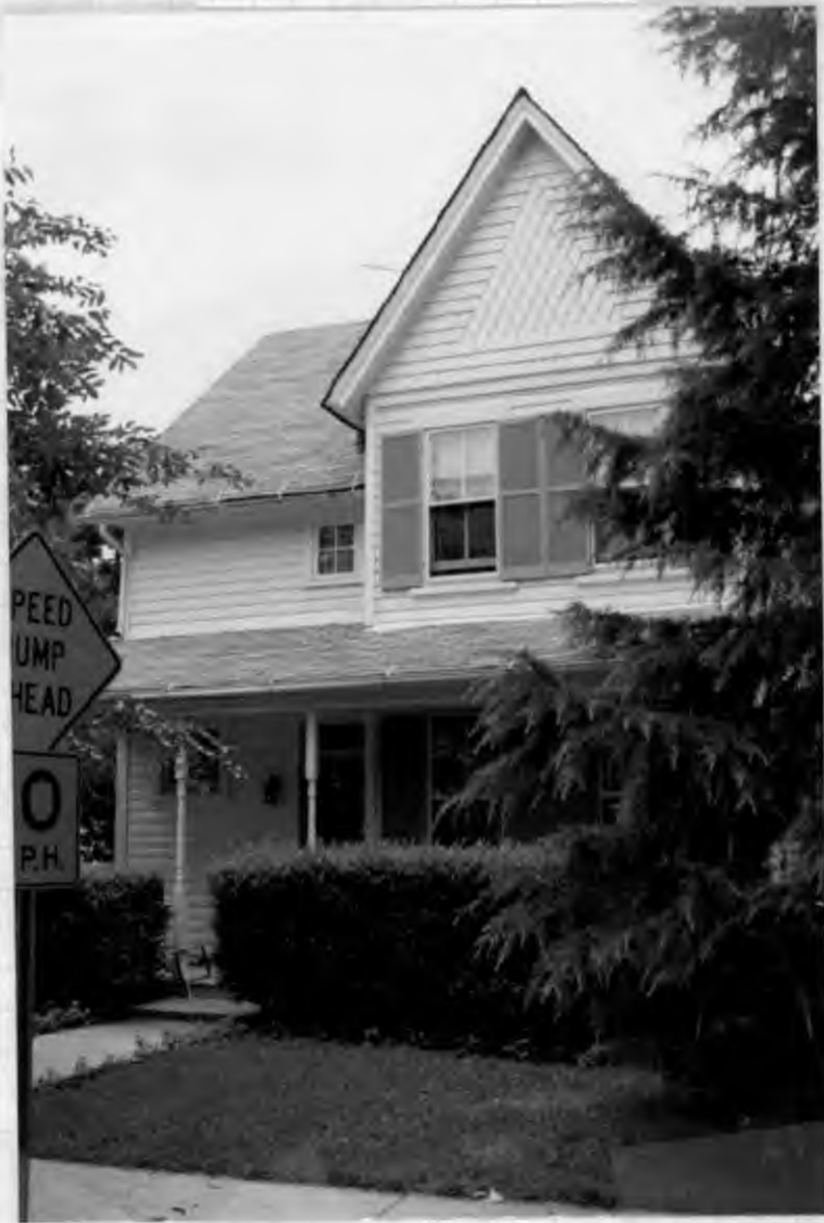
FRONT OF 10314 ARMORY AVE (EAST SIDE)
