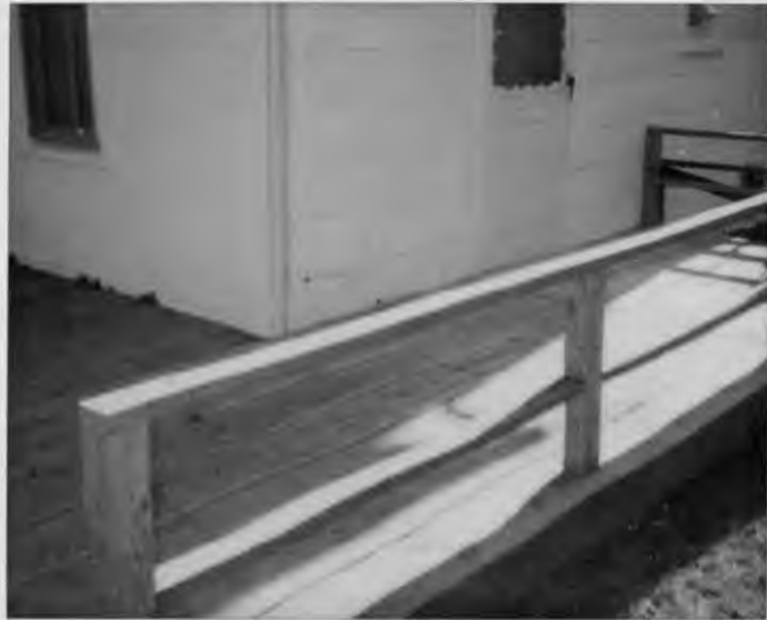
REAR DECK WEST FACADE
