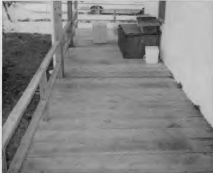
SIDE PORCH/DECK NORTH FACADE
