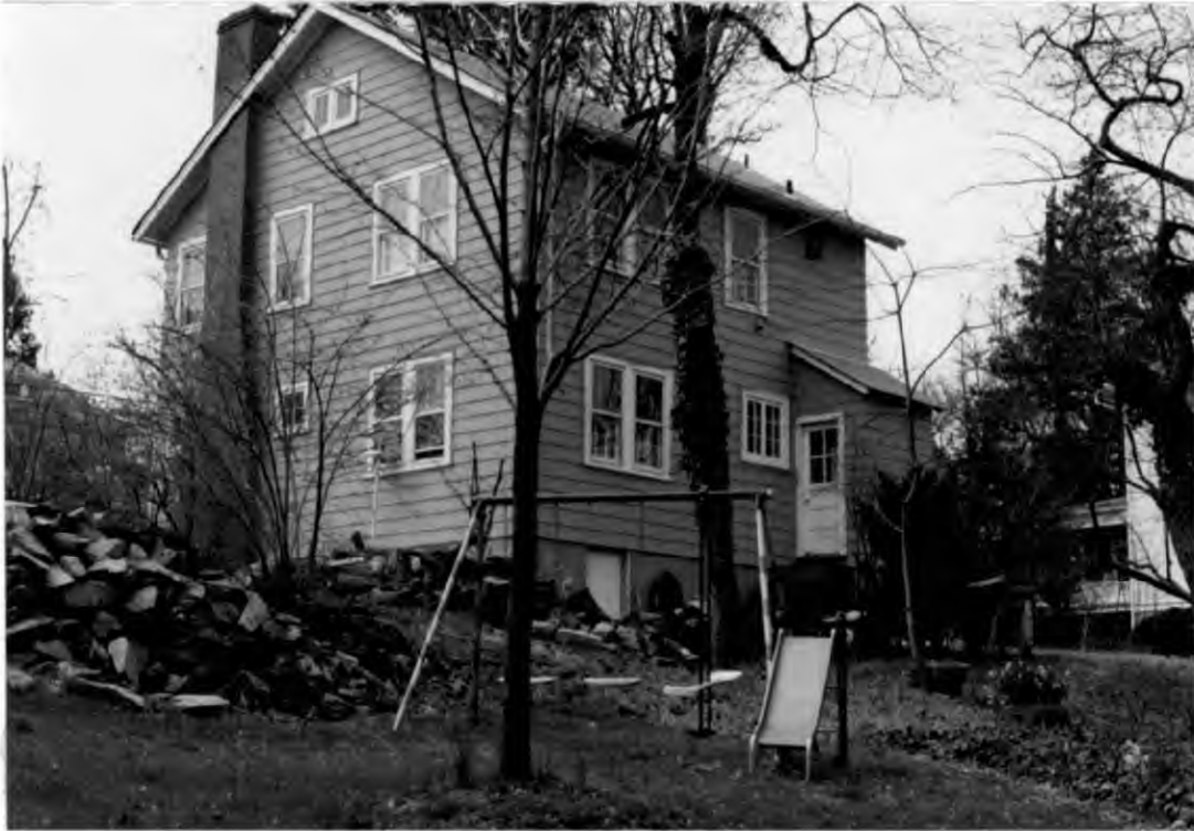
Rear and East Facades Viewed from 3915 Baltimore St.
