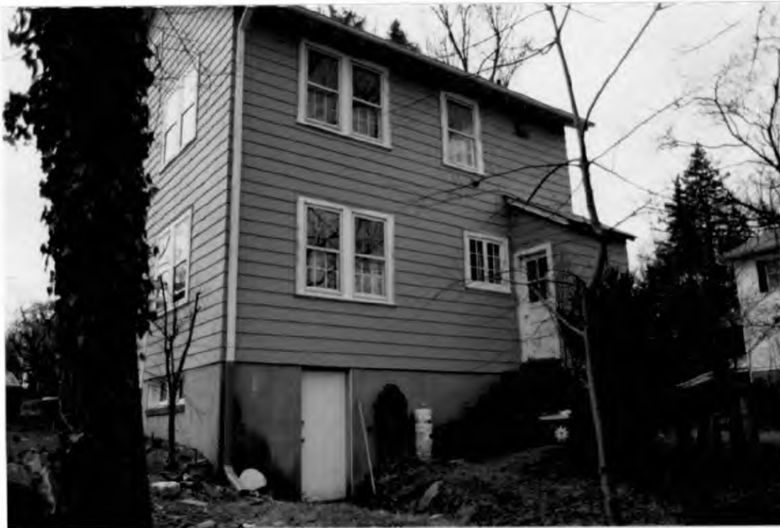
Rear and East Facades
