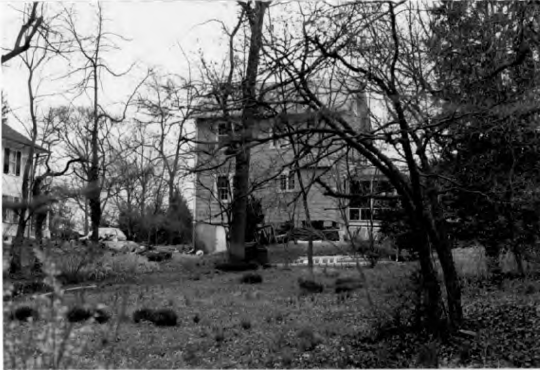
Rear Facade Viewed from 10311 Freeman Pl.
