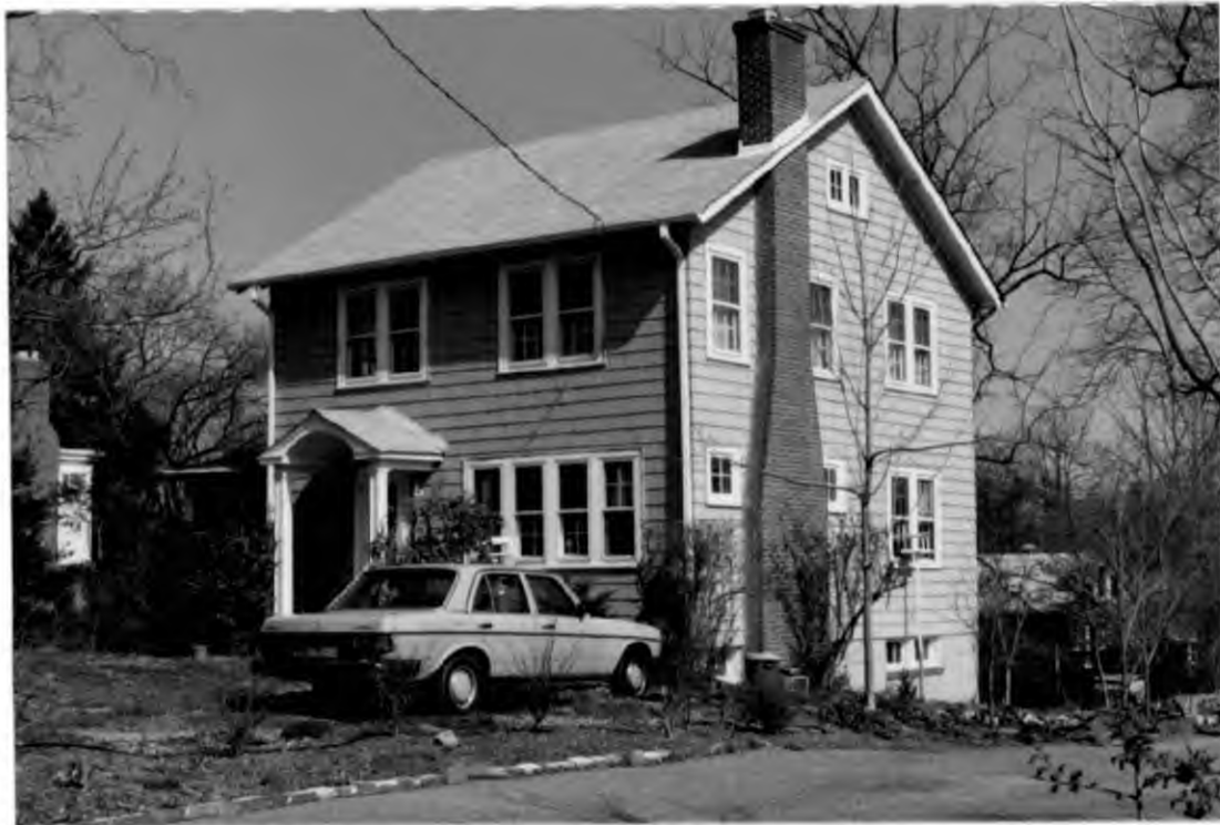
East Facade Viewed from Baltimore Street
