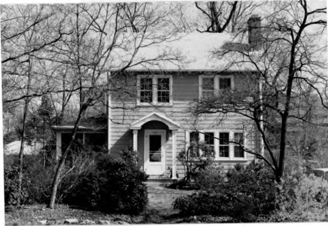
Front Facade Viewed from Baltimore Street
