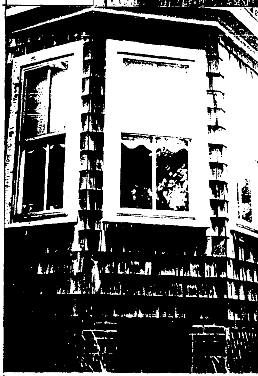
WINDOW & WINDOW TRIM
