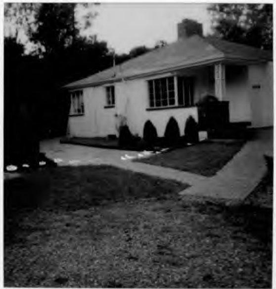
South side of house Fence separates parking area from side play area
