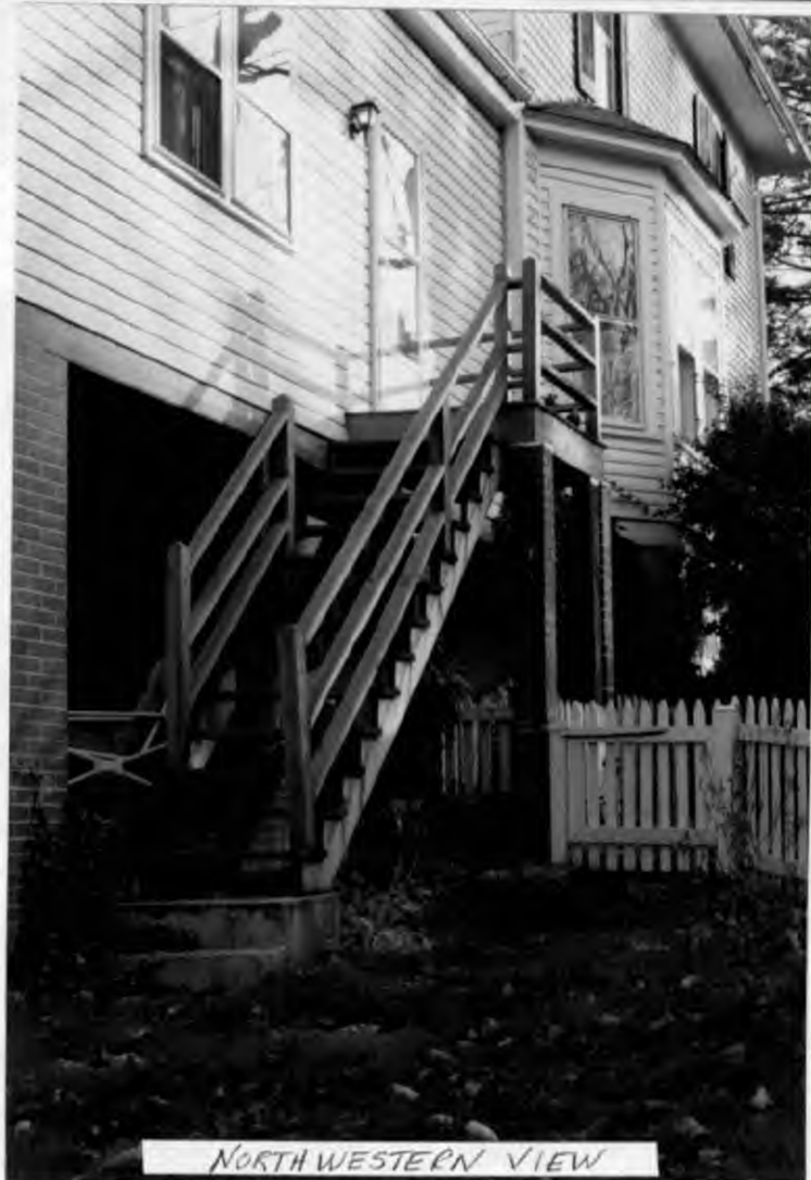
NORTH WESTERN VIEW
