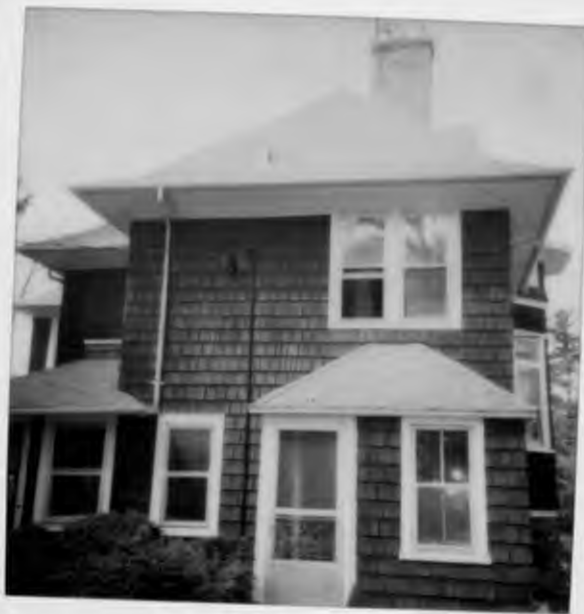
WEST (REAR) EXTEND ROOF, NEW WINDOWS @ BREAK RM
