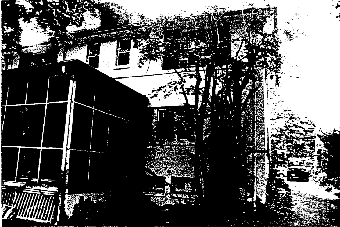
3. Northeast Corner Elevation
