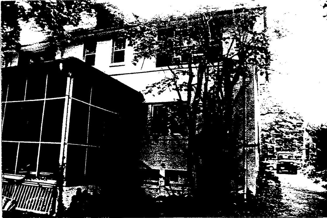
3. Northeast Corner Elevation
