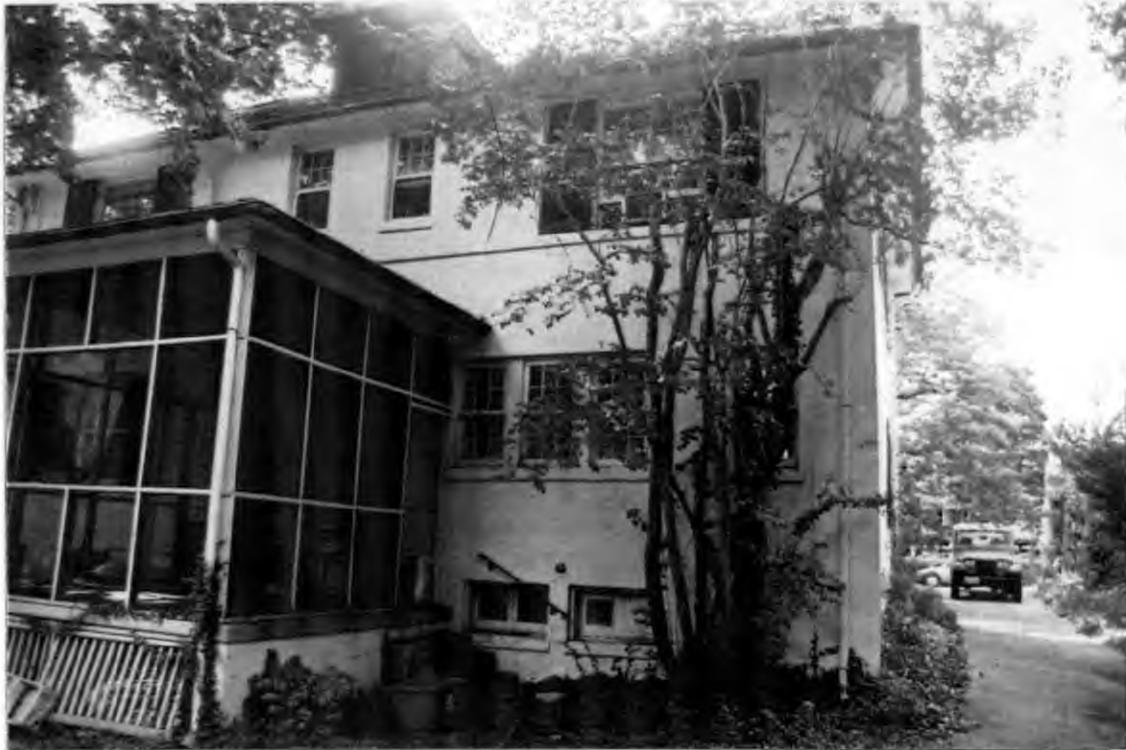
3. Northeast Corner Elevation
