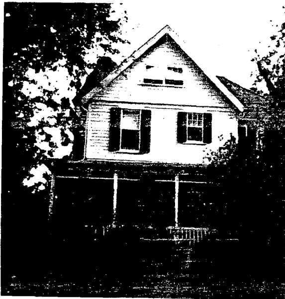
10216 KENSINGTON PKWY. NORTH FACADE
