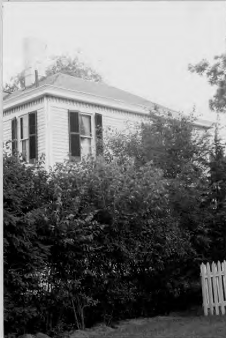
3. NORTHWEST CORNER - WEST ELEVATION
