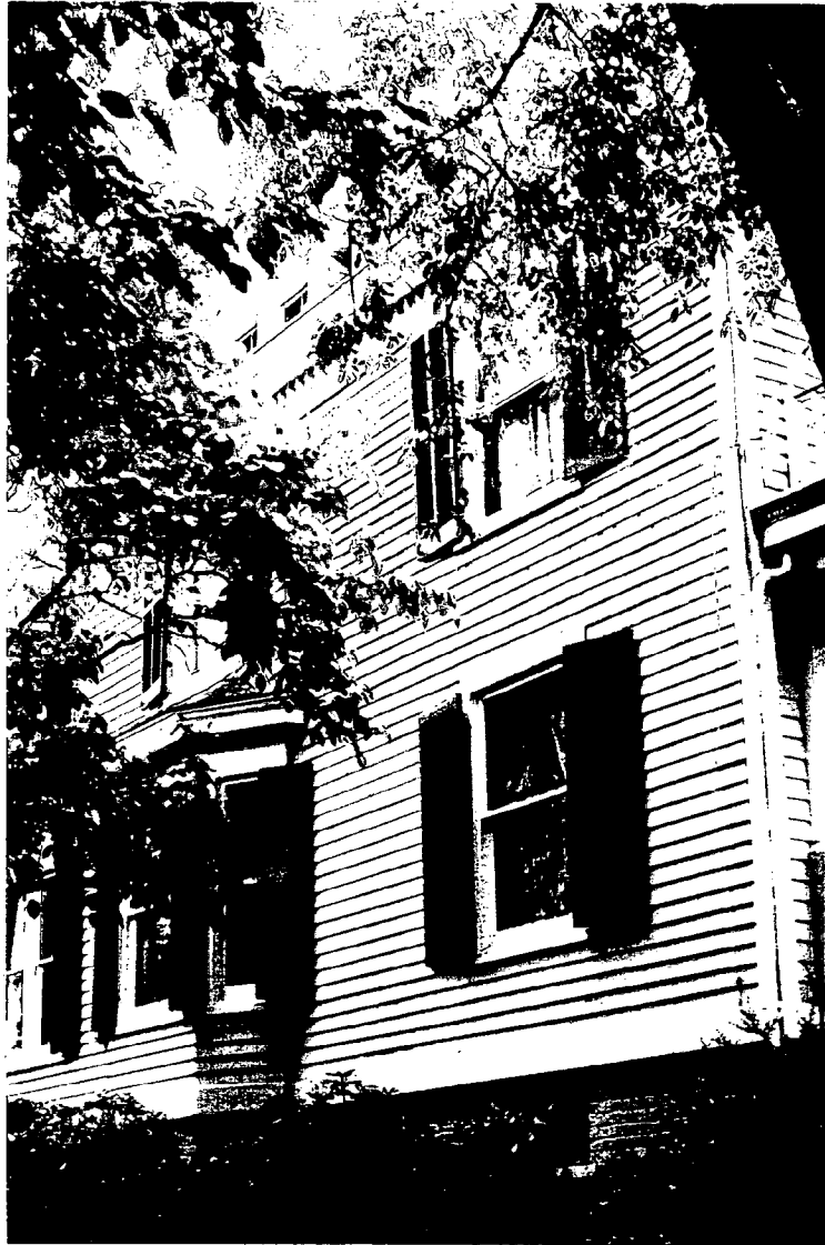
5. SOUTHEAST CORNER - PARTIAL SOUTH EL
