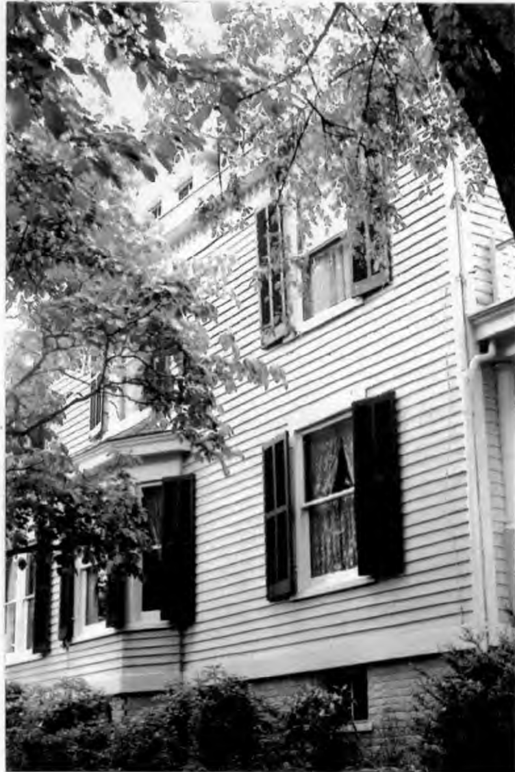
5. SOUTHEAST CORNER - PARTIAL SOUTH EL
