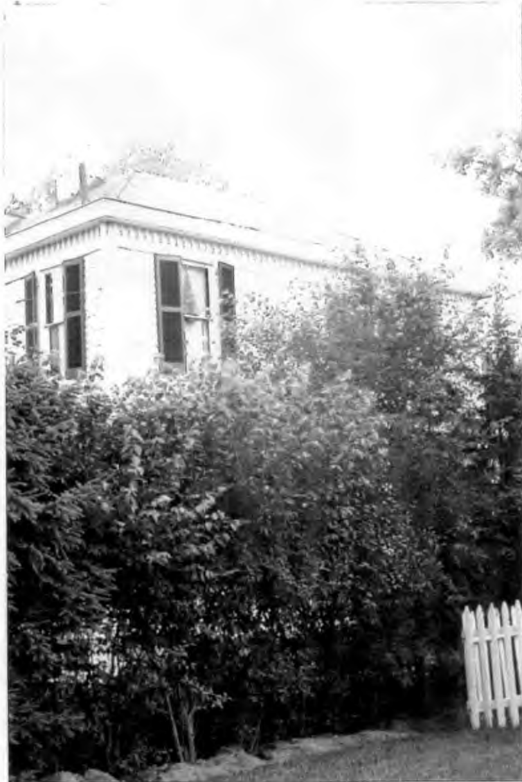
3. NORTHWEST CORNER - WEST ELEVATION
