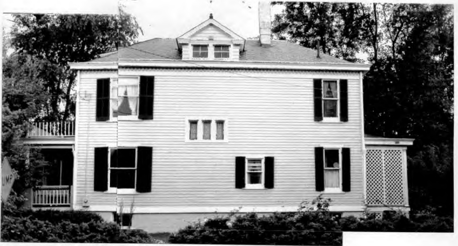
2. NORTH ELEVATION — WARNER STREET
