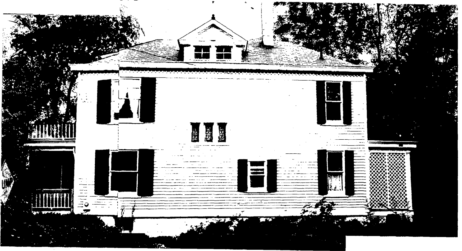
2. NORTH ELEVATION - WARNER STREET
