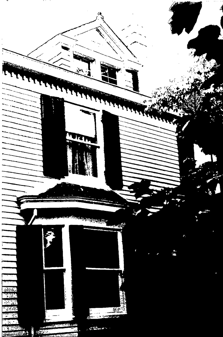
4. SOUTHWEST CORNER - PARTIAL SOUTH ELE
