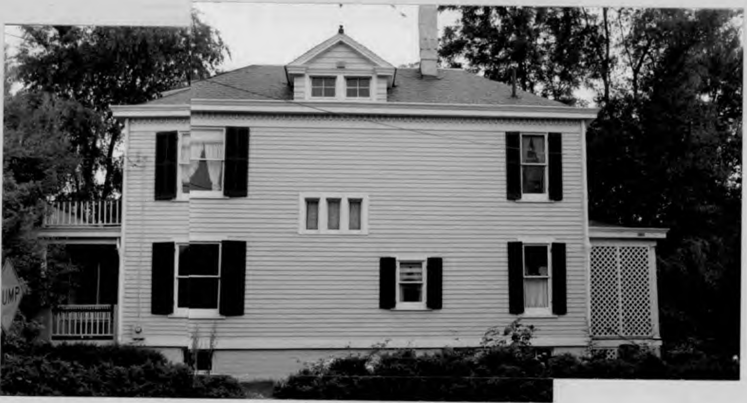
2. NORTH ELEVATION — WARNER STREET
