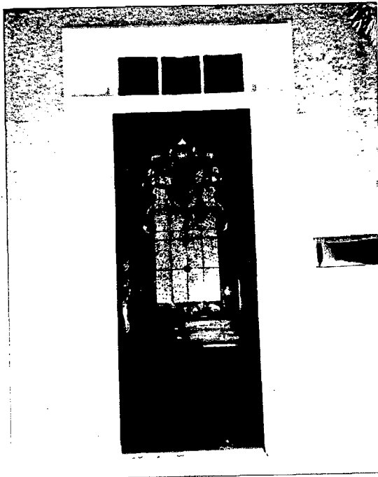
PHOTO TAKEN FROM EXTERIOR
