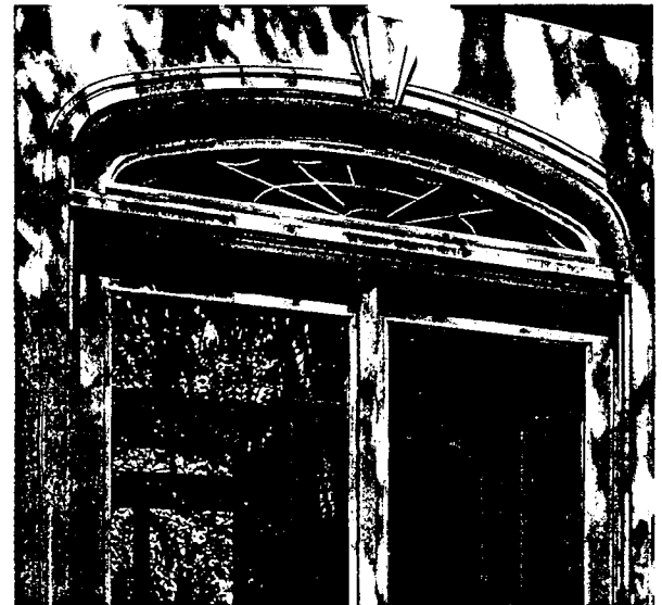
Elliptical Transoms were used over The Atrium Doors for this patio enclosure in Dayton, OH.
